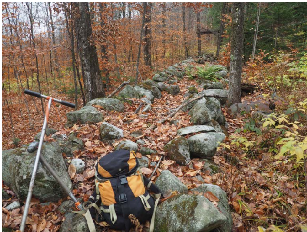
Figure 14. Stone wall composed almost entirely of granite. This one was constructed by building two parallel walls of granite boulders about three feet apart and filling the center with smaller rocks.
