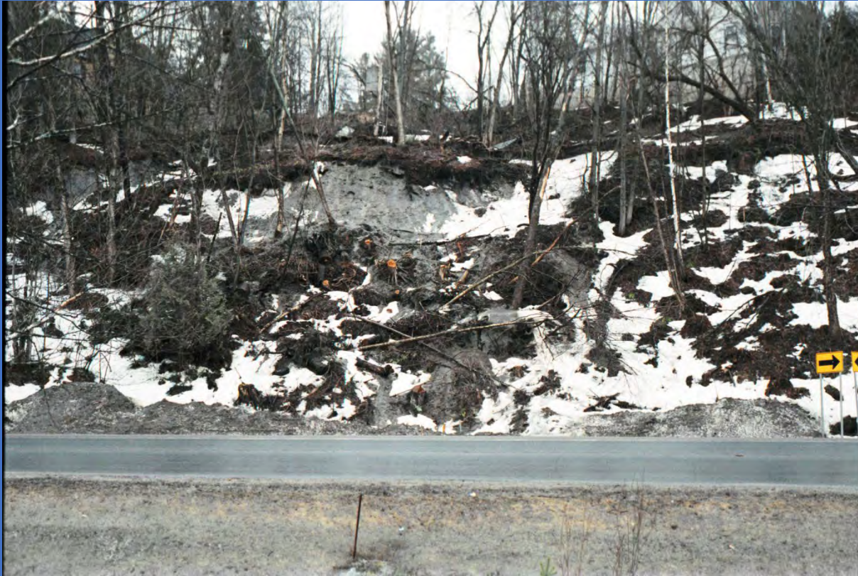
April, 2004. Looking up at slide from Vt. Route 15 prior to first slide across road in 2004. Note slide scarps. Some trees have been cut.
