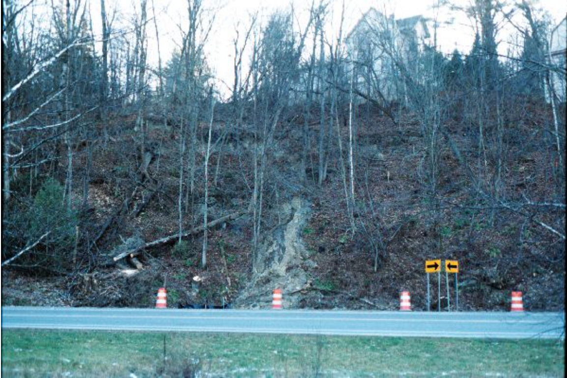
Figure 2. Landslide viewed from below. View looking south-southeast from motel parking lot on far side of Route 15. November 10, 2003.
