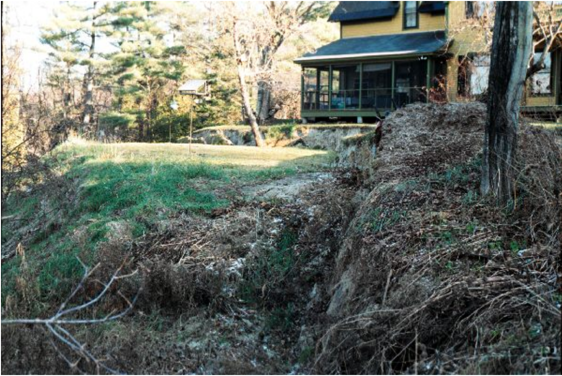
Figure 8. View looking east along fracture surface in artificial fill at Holmes residence. November 10, 2003.
