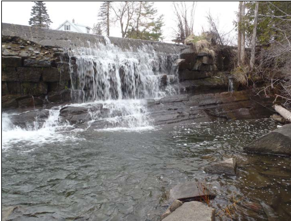
Figure 8. Ledge of phyllite of the Gile Mountain Formation exposed at the base of dam. Same site as Figure 7.
