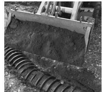
2. Backfill the trench.
