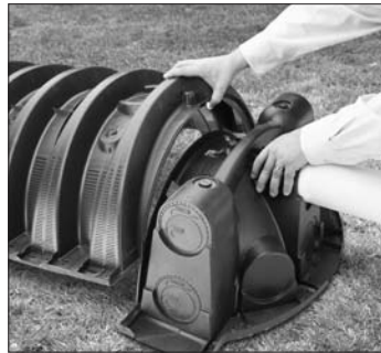
2. Place first chamber onto endcap.
