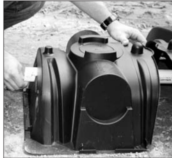
Lateral pipe through endcap.
