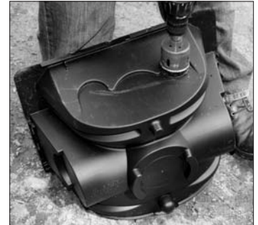
2. Drill pressure pipe hole.
