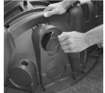
2. Pull tab on tear-out seal.
