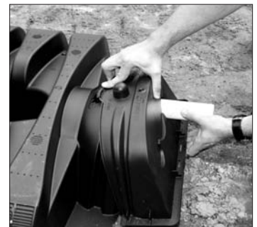
4. Place endcap over inlet end.
