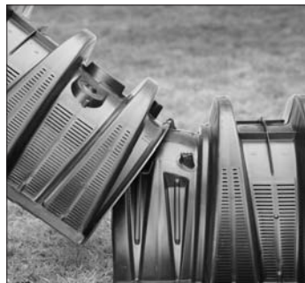
3. Connect the chambers.
