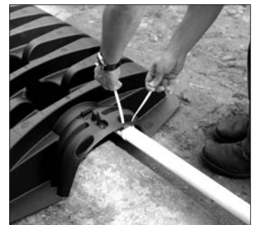
5. Secure pressure pipe.
