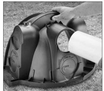
5. Insert inlet pipe.
