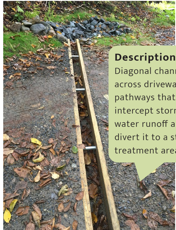
<Water bars, ^Open-top culvert and rock apron.
