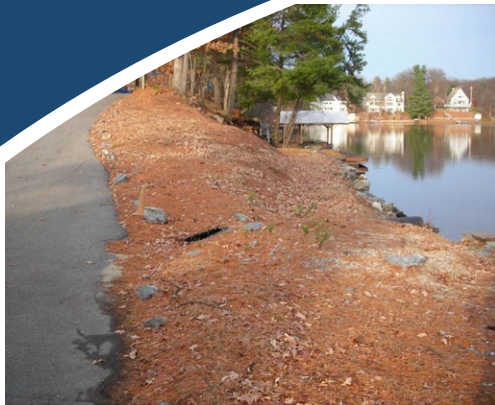
Before: drainage pipe conveys road runoff directly into Lake Shirley, MA.
