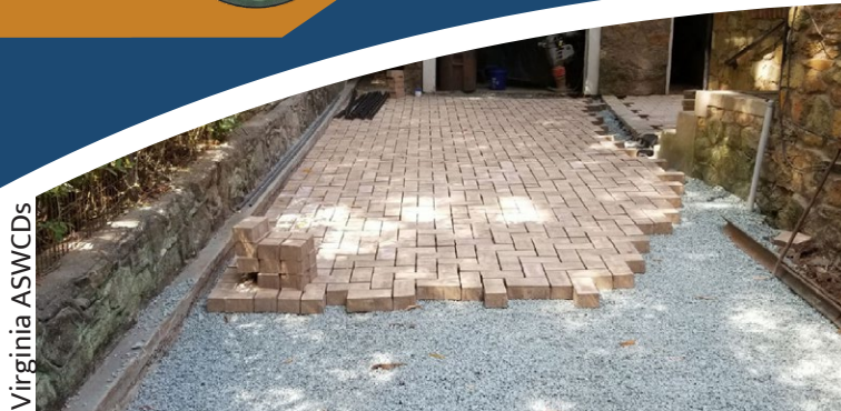
Laying interlocking permeable paver blocks.
