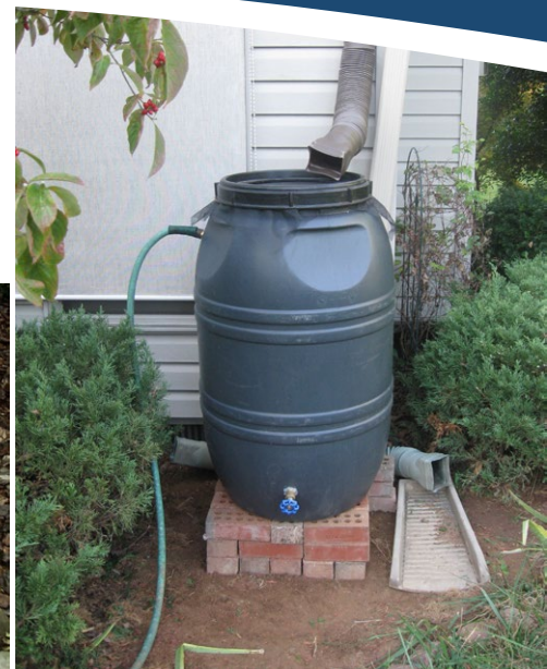
A rain barrel with gutter extension and splash pad for winter use.
