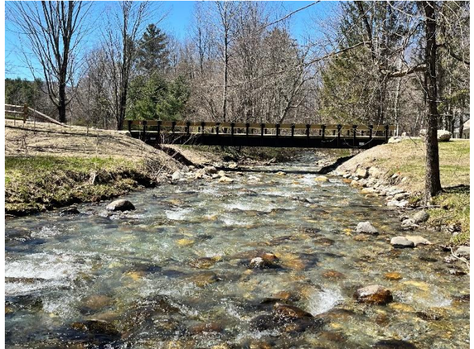
Figure 18: Before (left) and after (right) of a barrier removal and river channel restoration project on the Mettawee River in Dorset, Vermont. A concrete sill under a bridge created a large scour pool and severe bank erosion downstream of the structure. The sill was removed, and the bridge was widened to reduce further erosion. A support in the middle of the bridge was also removed, restoring 300 feet of the stream channel. Additionally, the upstream, river right, floodplain bench was lowered and a flood chute added so the river can better flow onto its floodplain when needed. The project was implemented by Trout Unlimited and funded with Clean Water Fund dollars administered through the South Lake Champlain CWSP's Water Quality Restoration Formula Grant. The Rutland Regional Planning Commission serves as the CWSP for South Lake Champlain basin in collaboration with Poultney-Mettowee Natural Resources Conservation District. Additional funding for the project was provided by the Lake Champlain Basin Program, U.S. Fish and Wildlife Service, U.S. Forest Service, and a private donor. Work was completed in the fall of 2023.
