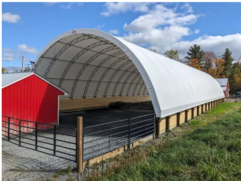
Figure 16: A barnyard improvement and cover was installed through the Best Management Practices (BMP) Program to reduce agricultural runoff to an adjacent stream from the farm's outdoor livestock area in the Connecticut River Watershed. Farms that are certified organic under the National Organic Program standards are required to ensure livestock have access to the outdoors every day. Covering those areas to prevent rainwater from mixing with animal waste can be an effective tool for reducing runoff and improving water quality on farms, especially during the winter months.
