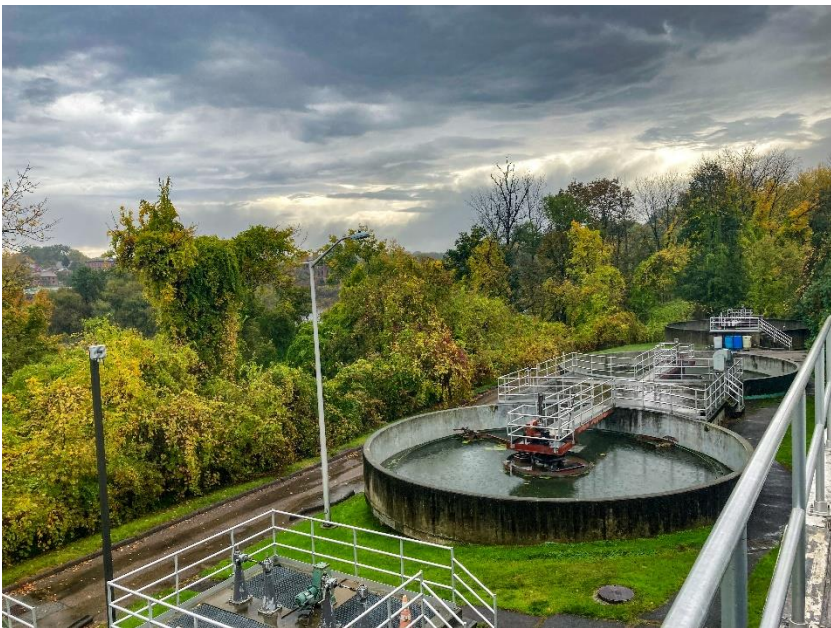
Figure 20: One of three wastewater treatment facilities operated by the City of Burlington. The city has partnered with the State of Vermont to finance several municipal wastewater treatment facility improvements and combined sewer overflow abatement projects. Financing this work has been possible in part by the low-interest loans available through the Clean Water State Revolving Fund.
