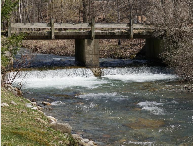
Figure 18: Before (left) and after (right) of a barrier removal and river channel restoration project on the Mettawee River in Dorset, Vermont. A concrete sill under a bridge created a large scour pool and severe bank erosion downstream of the structure. The sill was removed, and the bridge was widened to reduce further erosion. A support in the middle of the bridge was also removed, restoring 300 feet of the stream channel. Additionally, the upstream, river right, floodplain bench was lowered and a flood chute added so the river can better flow onto its floodplain when needed. The project was implemented by Trout Unlimited and funded with Clean Water Fund dollars administered through the South Lake Champlain CWSP's Water Quality Restoration Formula Grant. The Rutland Regional Planning Commission serves as the CWSP for South Lake Champlain basin in collaboration with Poultney-Mettowee Natural Resources Conservation District. Additional funding for the project was provided by the Lake Champlain Basin Program, U.S. Fish and Wildlife Service, U.S. Forest Service, and a private donor. Work was completed in the fall of 2023.
