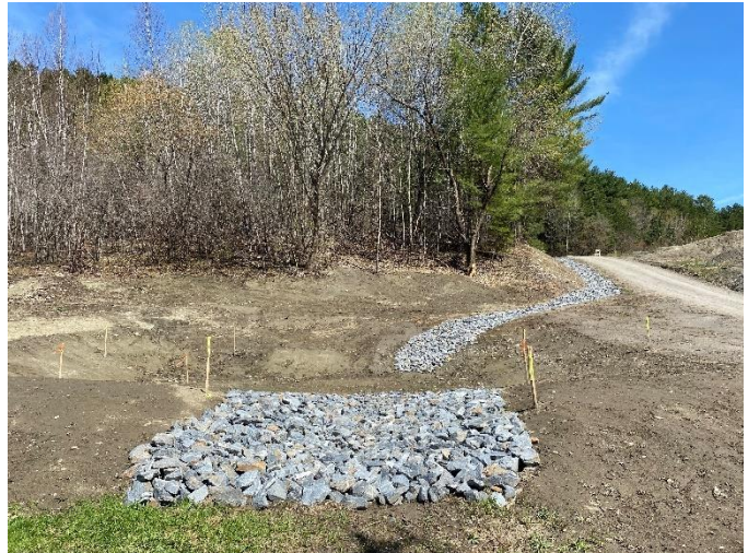
Figure 19: Before (left) and after (right) of a road and parking area stormwater erosion control project. The project area was identified as a high priority in the Stormwater Master Plan for the town of St. Johnsbury, Vermont. The designed practices manage almost 18 acres of impervious surface. The project was developed by the Caledonia County Natural Resources Conservation District (NRCD) with support from a Project Development Block Grant administered by the
