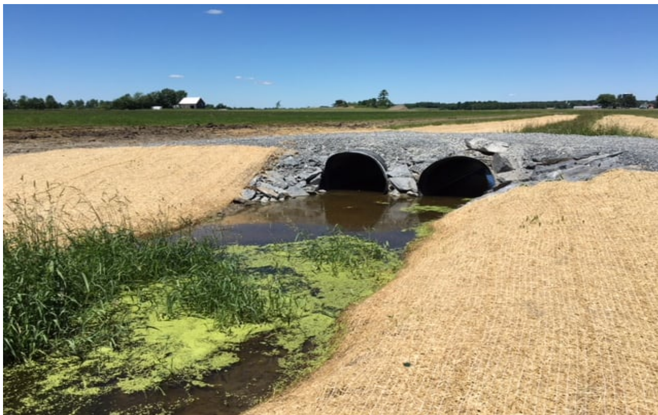
Figure 18. Two-tiered ditch on farmland in the Rock River watershed
