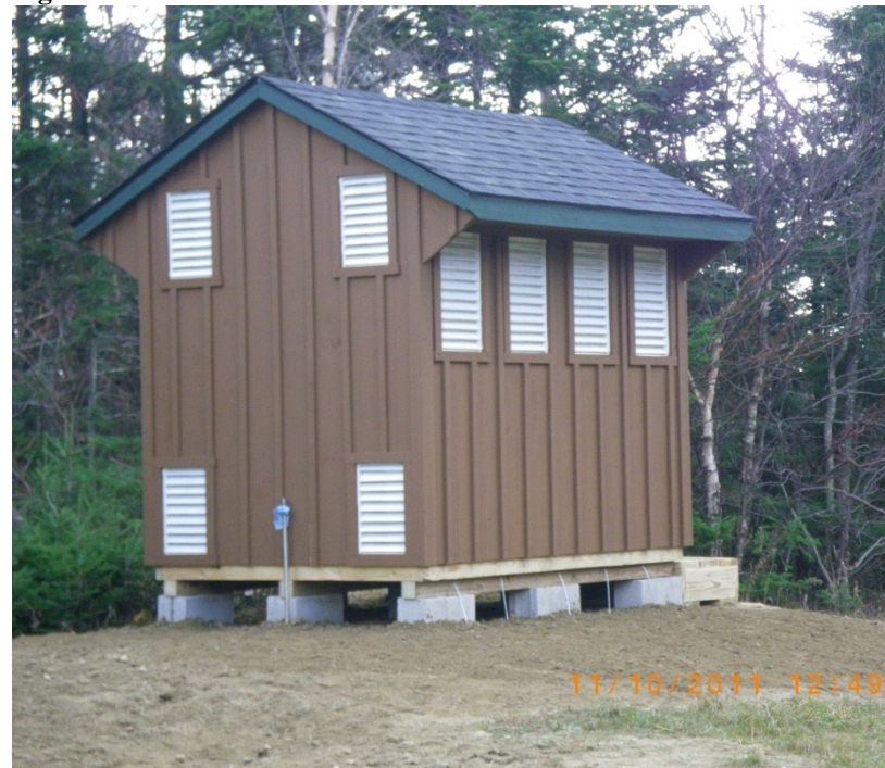
Figure 7 – View of Monitor Location
