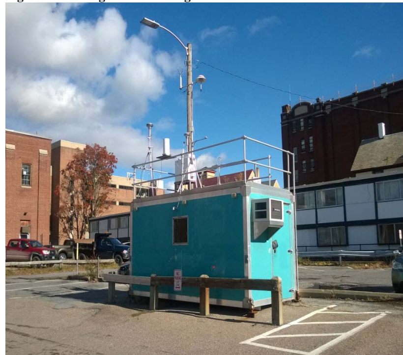
Figure 3– Burlington Monitoring Shelter
