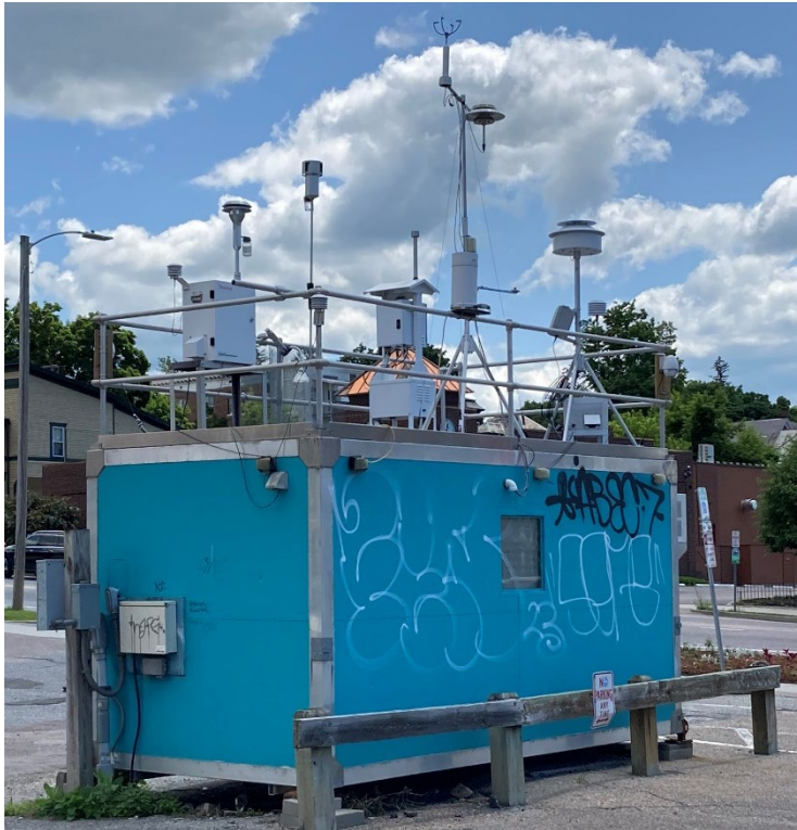
Figure 5 – Burlington Monitoring Shelter
