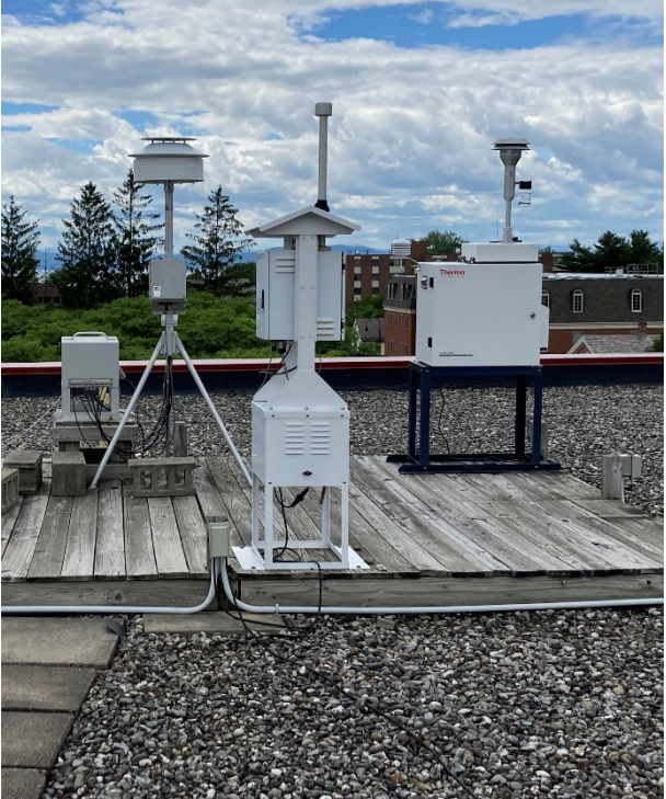
Figure 7 – Zampieri Building Sampling Platform
