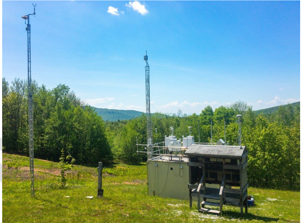
Figure 11 – Underhill IMROVE Shelter & Trailer
