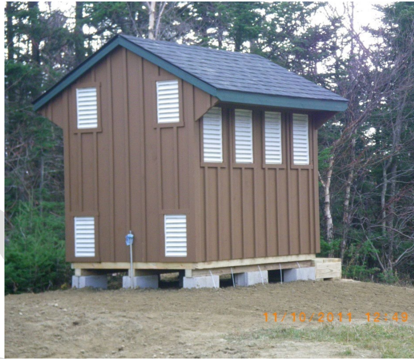
Figure 13 – Mount Snow Monitor Shelter
