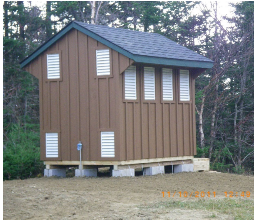
Figure 13 – Mount Snow Monitor Shelter
