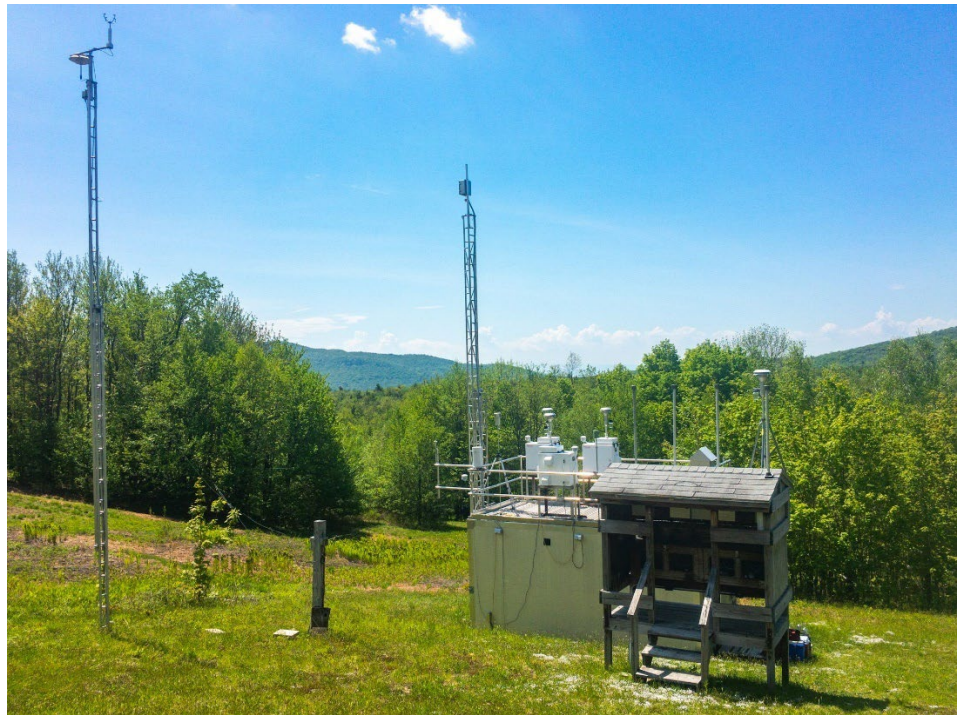
Figure 11 – Underhill IMROVE Shelter & Trailer
