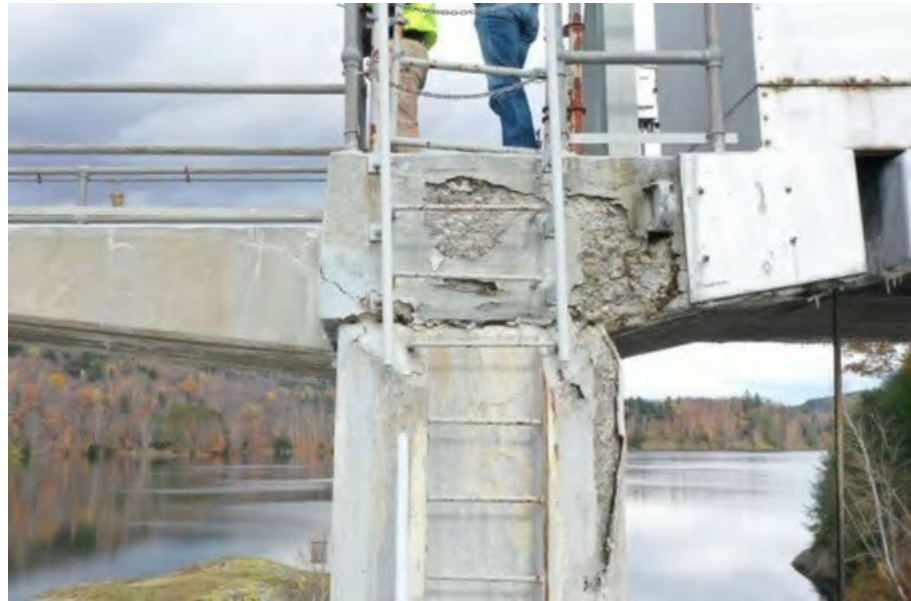
Fig. 2-2. Pier 4 – Hoistway Bridge Junction in 2022
