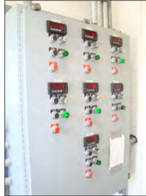
Gate Controls/ SCADA Systems
