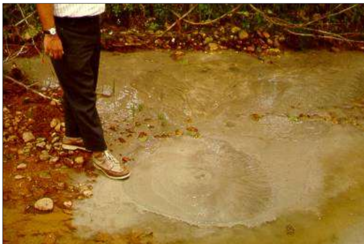
Embankment Seepage - Boil
