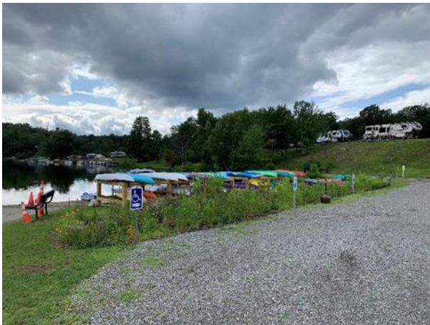
Photos from after the restoration project showing the bioretention area and native plants installed to slow and absorb stormwater before it reaches the lake.
