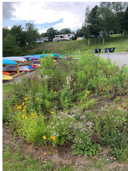
Photos from after the restoration project showing the bioretention area and native plants installed to slow and absorb stormwater before it reaches the lake.
