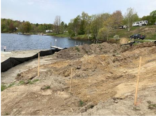
Photos from before and during the restoration process showing lawn area that went directly to the lake, with nothing to stop or slow rainwater coming off the driveway, parking lot, and lawn.
