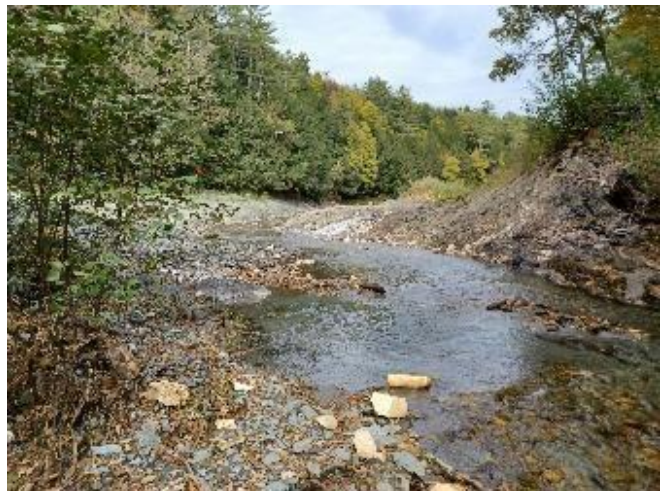
North Breton Brook after removal of the Pelletier Dam. Aquatic organism passage has been restored in this section of the brook and the river has space to move, allowing for natural channel evolution and reduction in erosive channelization.
