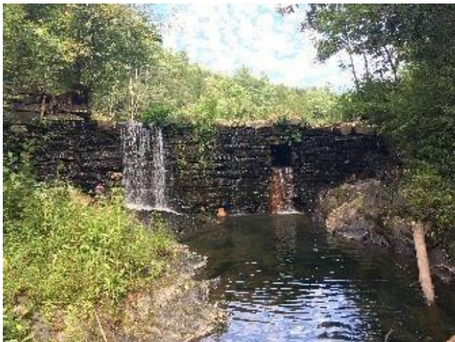
Pelletier Dam on North Breton Brook in Castleton, VT prior to removal.
