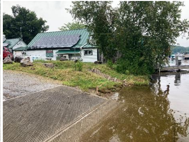
Before images of the Lake Dunmore Fish and Wildlife Access Area showing no drainage or buffer was present between the parking area and the lake.
