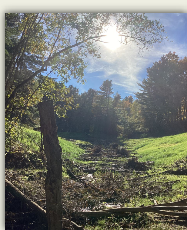
Dam removal and river & floodplain restoration
