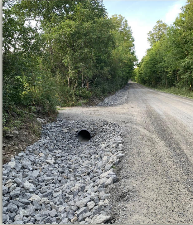
Road erosion mitigation projects
