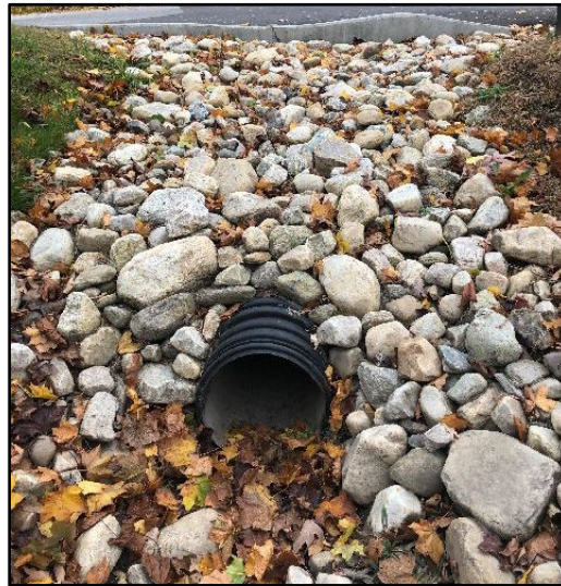
Example photo of Minor natural debris at the inlet.
