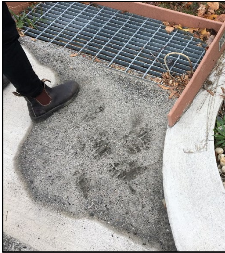
[Left] Example of Minor sediment accumulation at the inlet. [Right] Example of Major sediment accumulation at inlet.
