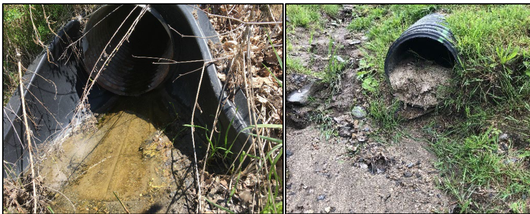
(Left) Example of outlet with Minor sediment accumulation. (Right) Example of Major sediment accumulation.
