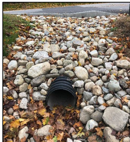
Example photo of the inlet to a stormwater practice.
