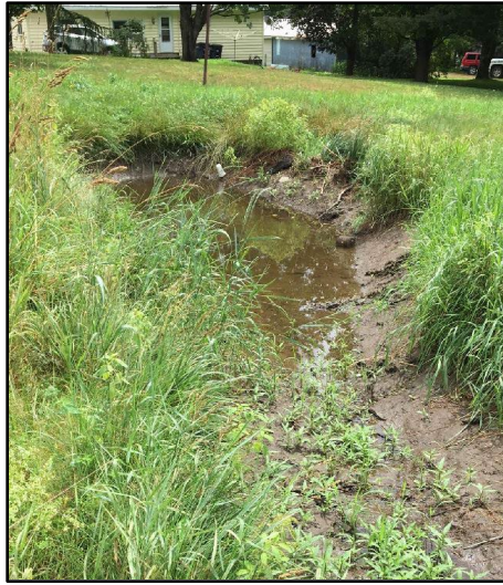
[Left] Example of >30%-50% pretreatment filled with sediment. [Right] Pretreatment forebay 100% full of sediment.
