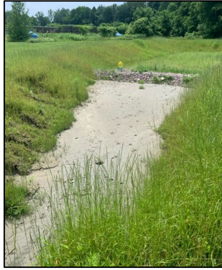
[Left] Example of >30%-50% pretreatment filled with sediment. [Right] Pretreatment forebay 100% full of sediment.
