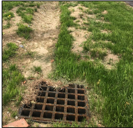
Example photo of Moderate erosion (Rill I).
