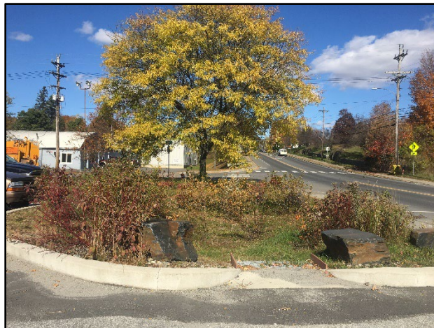
Example photo of a bioretention showing full extent of the practice.
