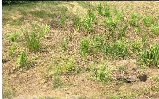
Photo example of 50-70% vegetative cover in a gravel wetland.
