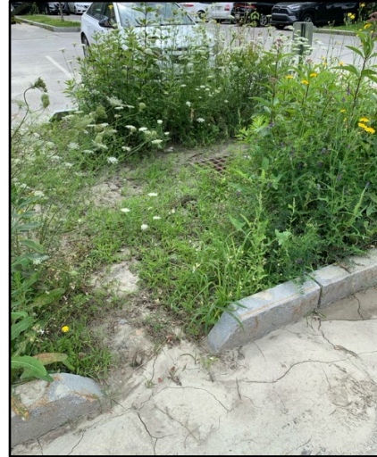
[Left] Example of Minor sediment accumulation at the inlet. [Right] Example of Major sediment accumulation at inlet.
