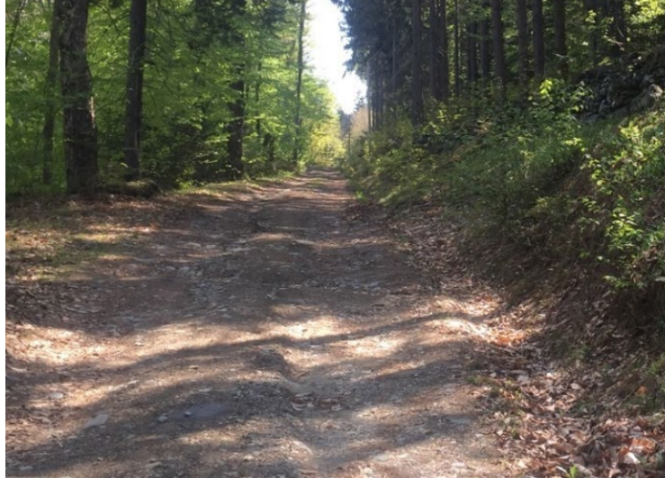
Figure 5. An example of a forested road constructed of native material with significant rutting.
