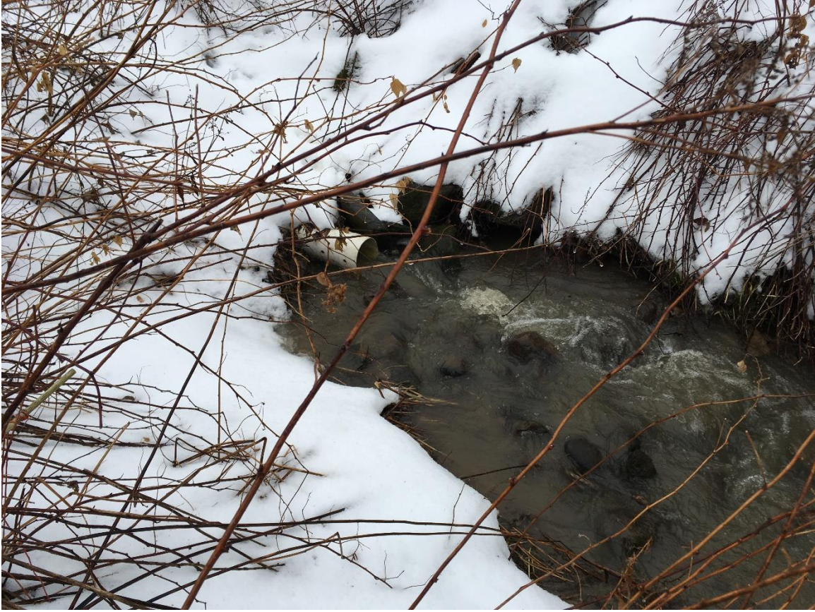
IMG_1722, Taken on 1-23-2018 by John D. E. Roberts. The photo depicts where the tile under the grassed waterway leading from the tiled field comes out by the cedar woods down near Lake Carmi. The water coming out of the tile has some mild sediment in it on this day.
