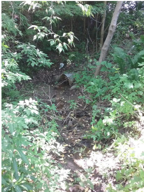
Wetland A, east side; intermittent stream at culvert inlet
