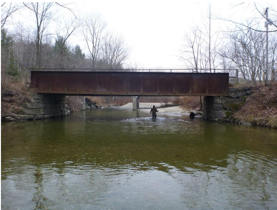
FIGURE 6-3: Railroad/Cambridge Greenway Bridge during low flow 12/6/12. Constricting abutments are shown (Source: FEA).
