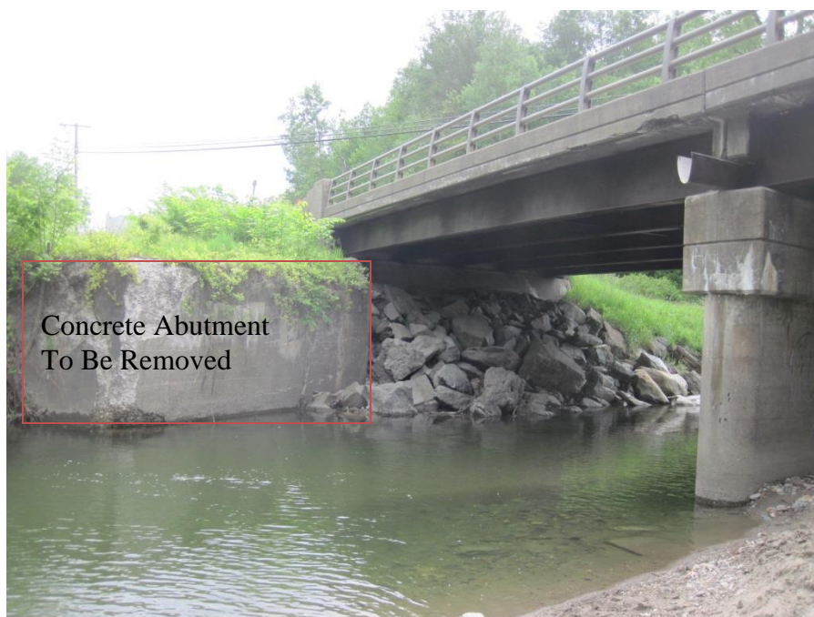
FIGURE 6-4: Old Route 15 abutment adjacent to Route 15 bridge, shown during low flow 6/6/2013. This concrete abutment is a constriction (Source: MMI).
