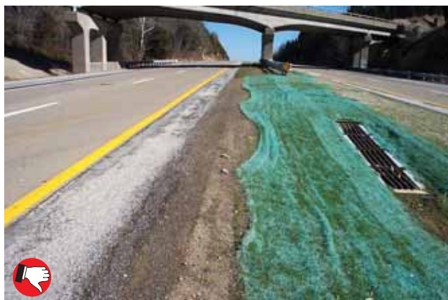
Good application of erosion control blanket to stabilize shoulder and protect storm drain, but too few staples used along the top edge. Trench in top edge of blanket on steep slopes.
