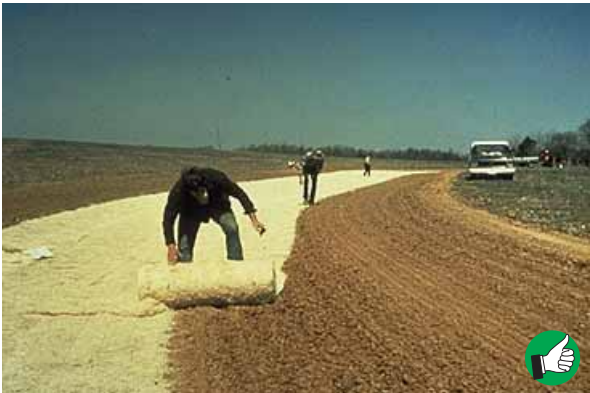
Blankets installed along stream banks or other short slopes can be laid horizontally. Install blankets vertically on longer slopes. Ensure 6 inch minimum overlap.
