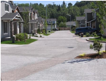
Figure 4_324-36. Pervious concrete roads in Sultan, WA (Source: Washington Aggregates and Concrete Association)
