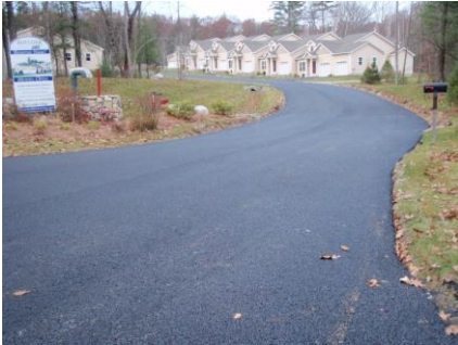
Figure 4_314-35. Porous Asphalt in a Low-Density Residential Area in Pelham, NH (Source: UNHSC)
