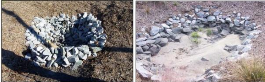
Figure 6-12. Plunge Pool Maintenance (NCDOT 2014)
