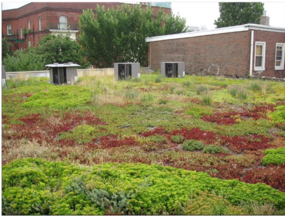
Figure 4-294-33. Example of extensive green roof, Philadelphia, PA (Source: UNHSC)
