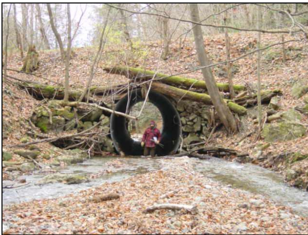
Beecher Hill Brook (T5.01B) culvert. Note aggradation forming bars and splitting flow upstream. Some erosion was noted downstream, although the downstream end falls onto ledge and boulders.
