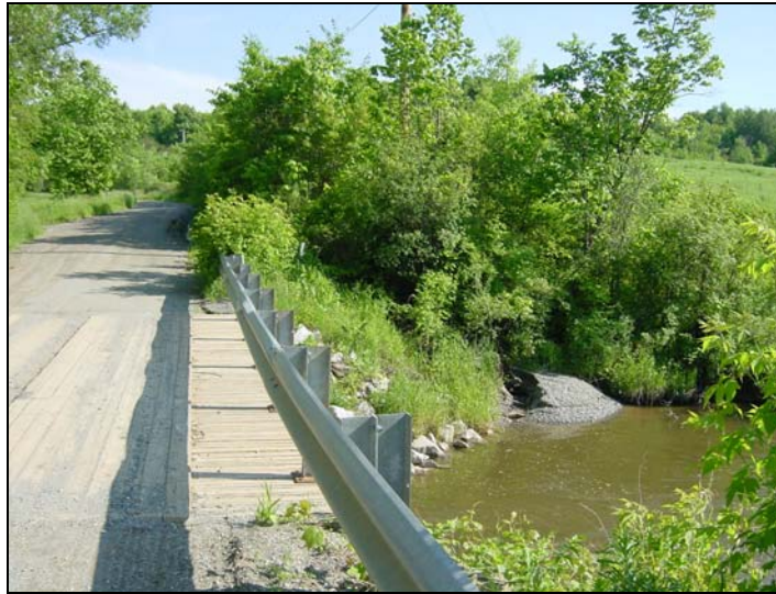
Leavensworth Road and bridge at M12 with large sediment deposit on the right where the road ditch meets the channel.
