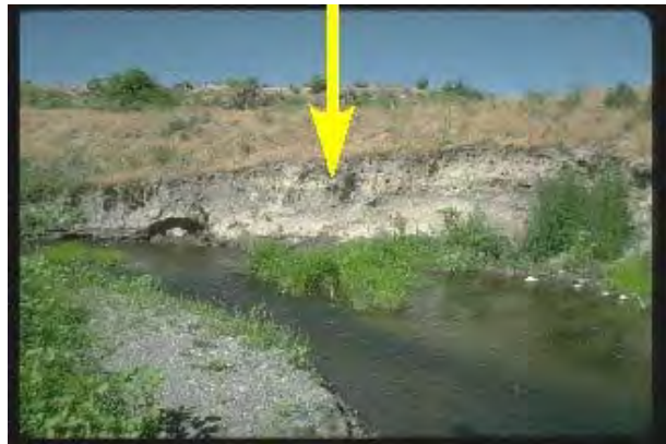
Figure 6.11B Poor bank stability
