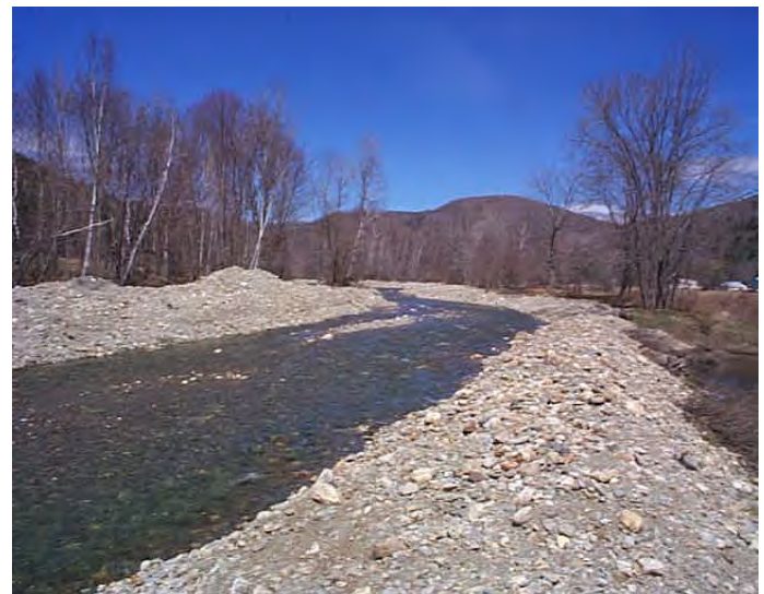
Figure 1.2 Berms built with river-dredged material.
