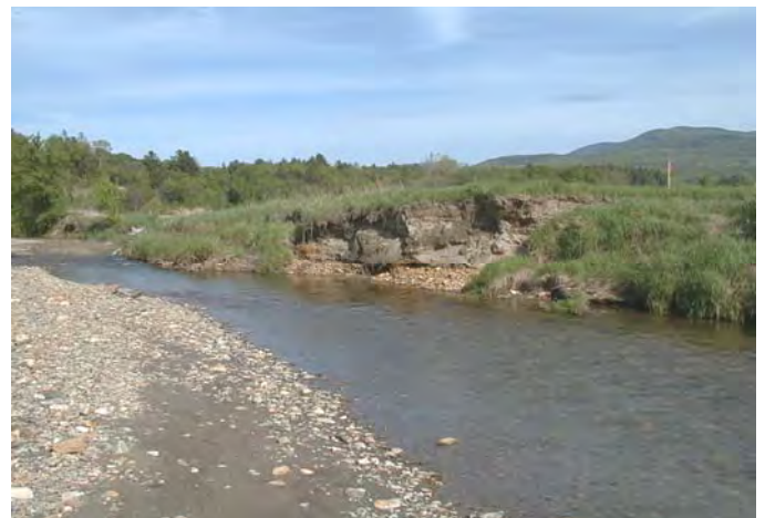
Figure 3.5 Slumped eroding bank.
