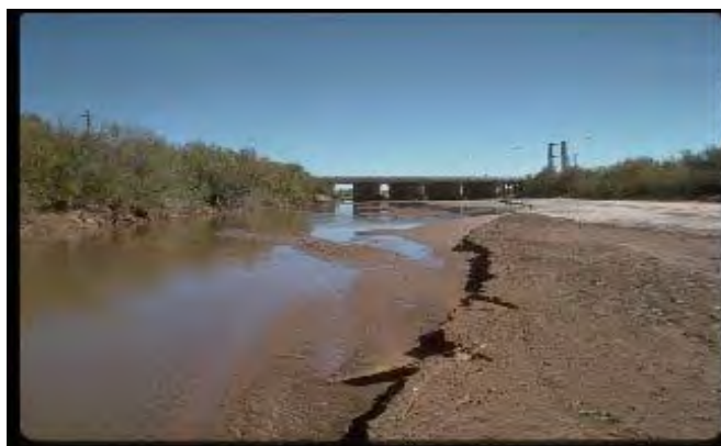
Figure 6.3B Poor pool substrate condition
