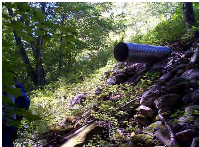
Figure 4.2 Roadway ditch stormwater culvert.
