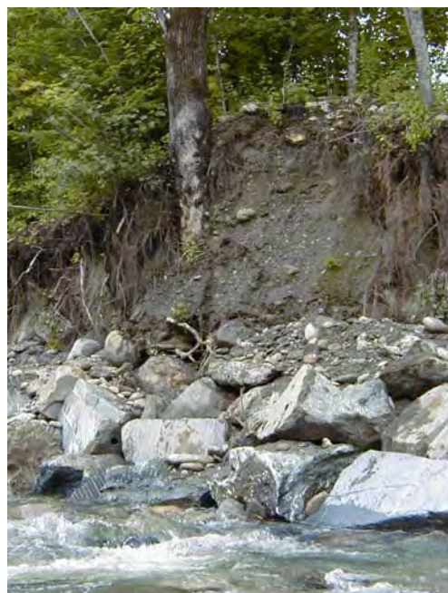
Figure 6.8C Example of berm and streambank armoring with stone wall. Dirt on top of stone wall is an old berm; note large tree growing in berm that was present before berm was constructed. Saplings on top of berm have grown up since berm was built several decades ago. Berm height above average water level is approximately 10 feet.
