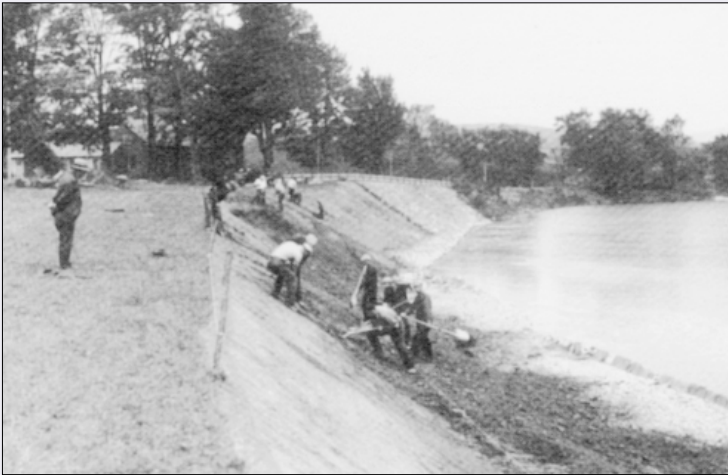
Bank shaping prior to installing soil bioengineering practices, Winooski River, September 1938
