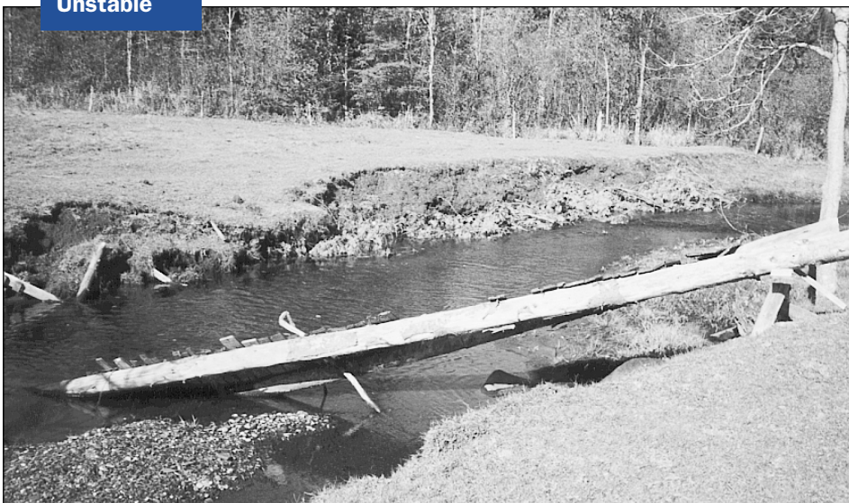
As banks erode and rivers widen, infrastructure such as this small bridge collapses.
