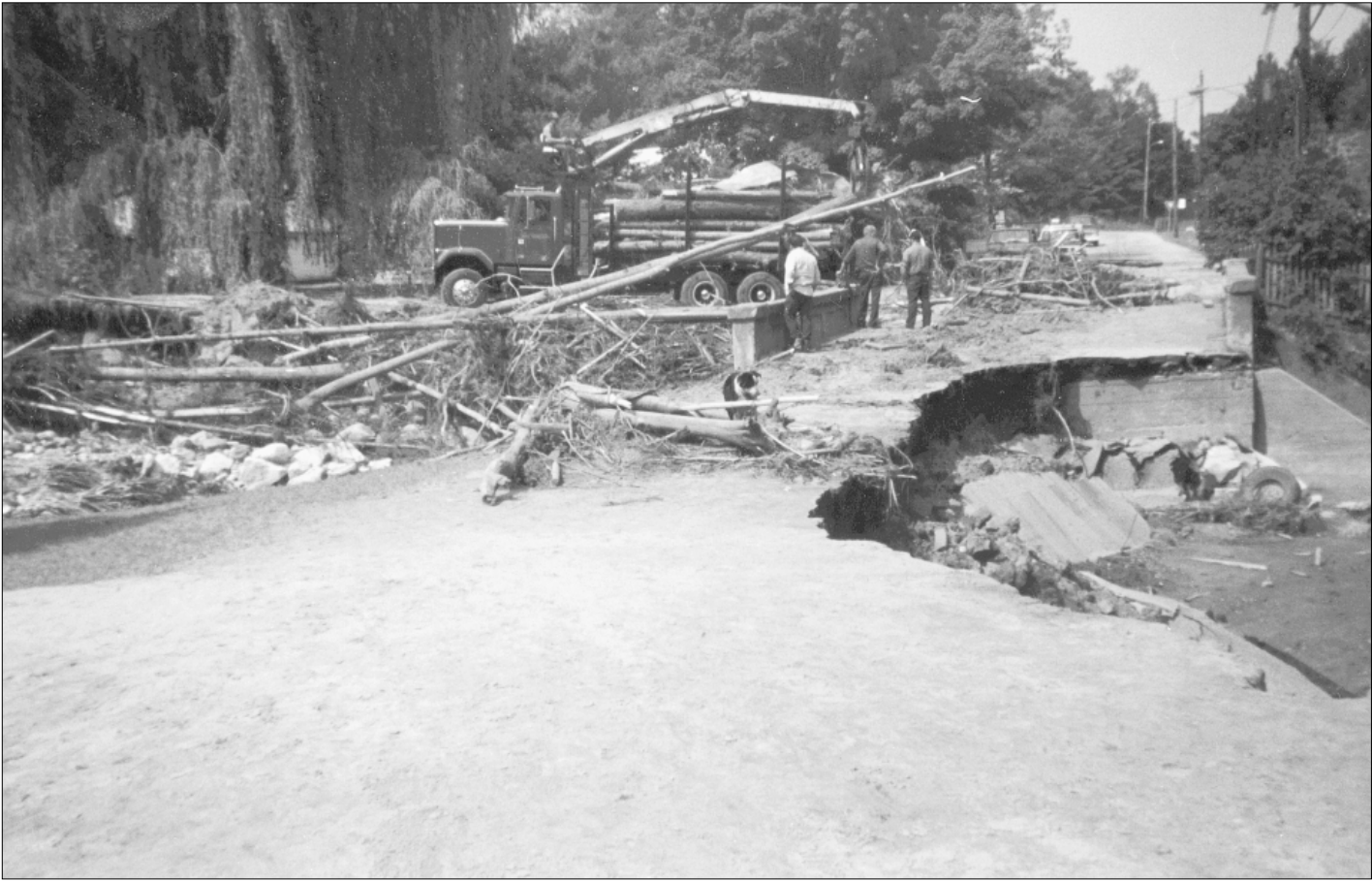
This road washed out during a flood on the Great Brook in Plainfield in 1990. This is an all-too-common event along rivers throughout Vermont.
