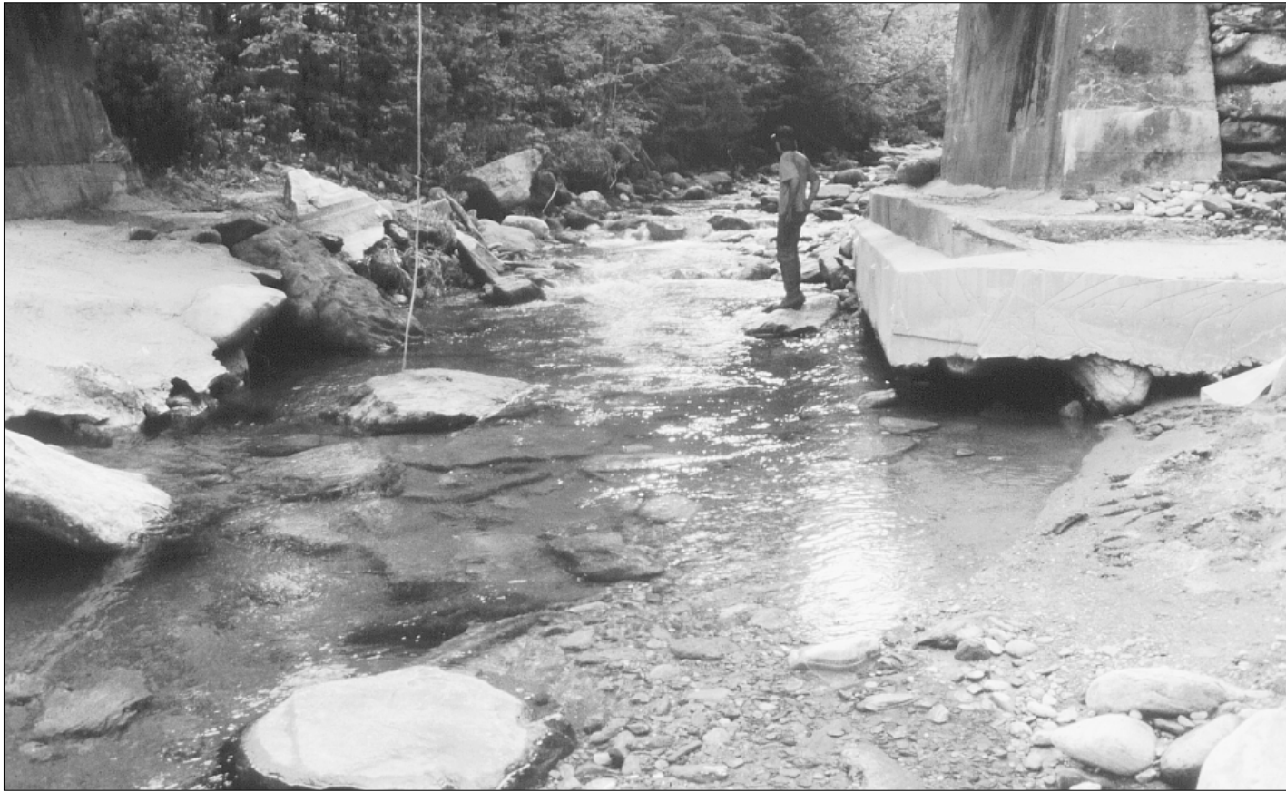
Vermont has many bridges that have been undermined as rivers have cut into the landscape in response to hydrologic changes in the watershed and modifications such as gravel mining or straightening of the stream channel. The Federal Highway Administration in 1995 wrote that federal funds are not available for bridges damaged by gravel mining.
