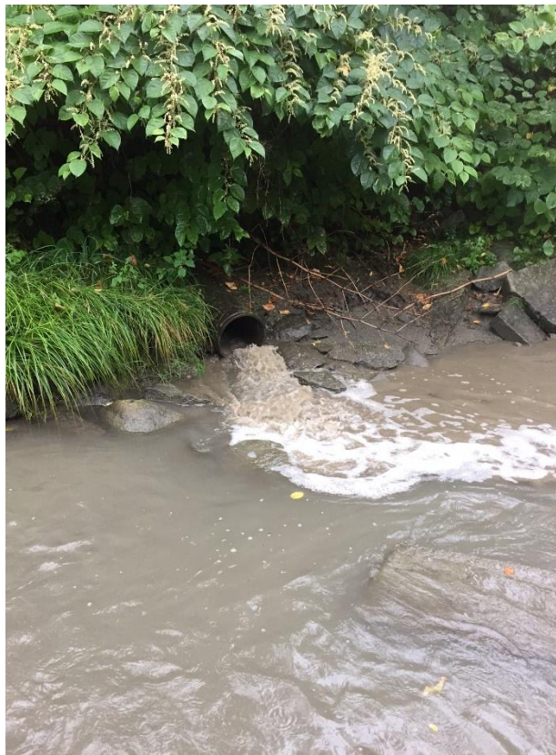
Photo 2 – Storm water flow directly entering the Jail Branch on Boynton Street in Barre City.
