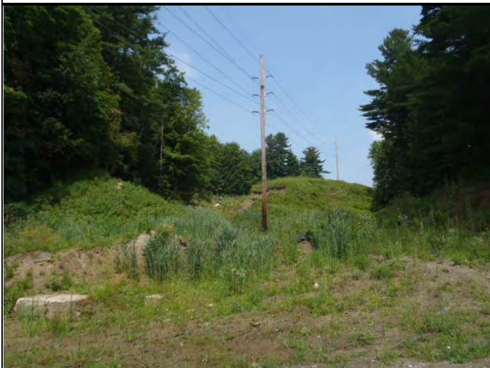
Photo 1. Landslide area from access road
