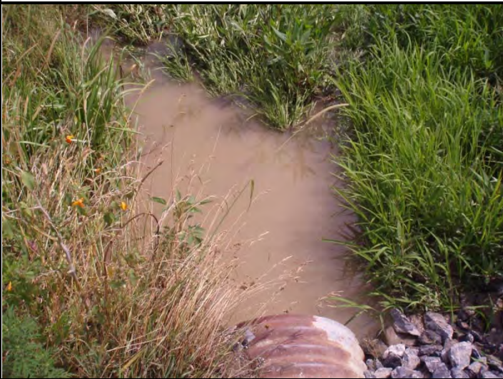
Photo 1. Upstream of farm road bridge
