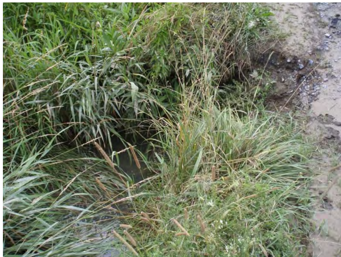
Figure 23. Undersized culvert under farm road. Erosion occurring from road surface as well as in scour pools at the upstream (shown) and downstream ends of the culvert.
