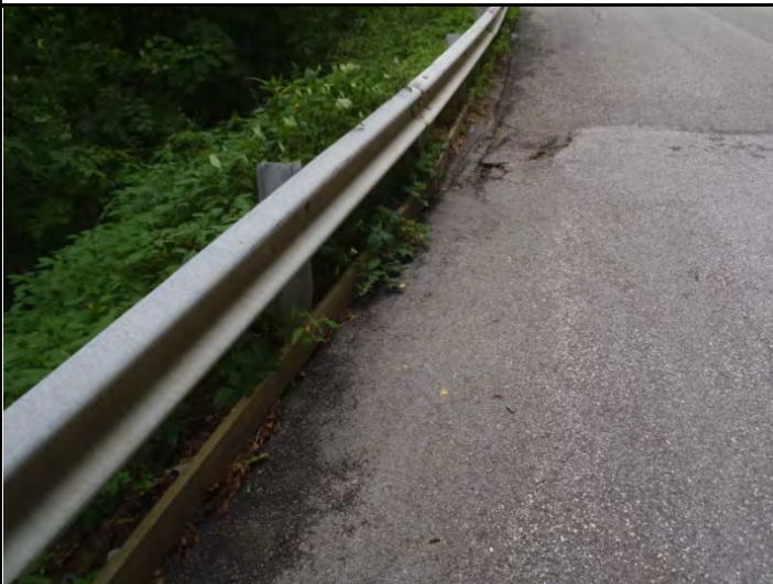
Photo 1. Erosion along roadside
