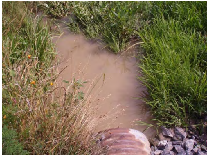
Figure 21. Scour pool at outfall from undersized culvert that carries unnamed Rock River tributary under farm road. Some rip rap has been placed by the landowner to address localized erosion around the culvert.
