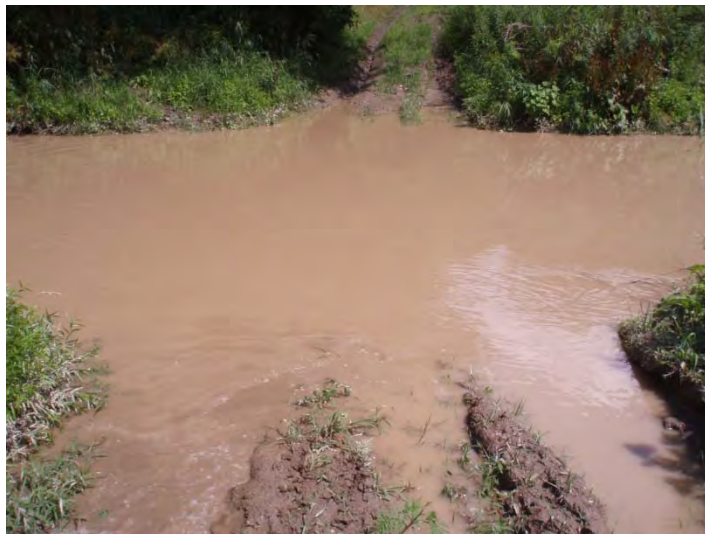
Figure 25. Unimproved farm road crossing, shown during high flow conditions. Significant ruts suggest landowner challenged to ford river during certain flow regimes.
