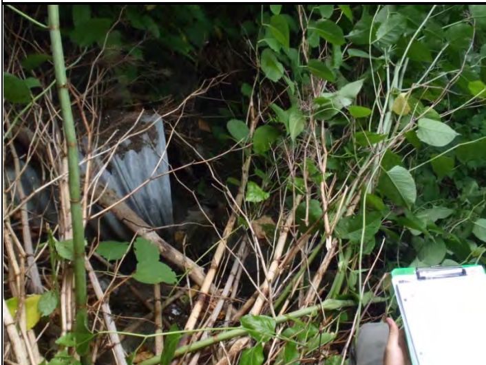
Photo 1. Outfall from under-road culvert
