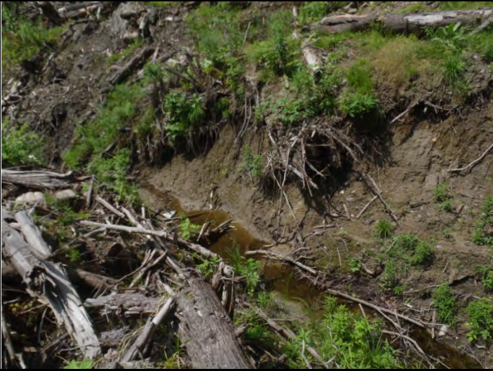
Photo 3. Channel dug by town to allow water flow
