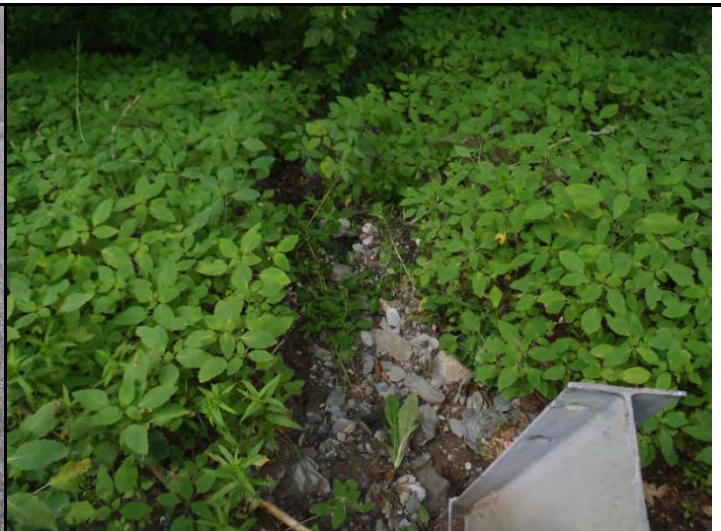
Photo 2. Blowout at the end of guardrail
