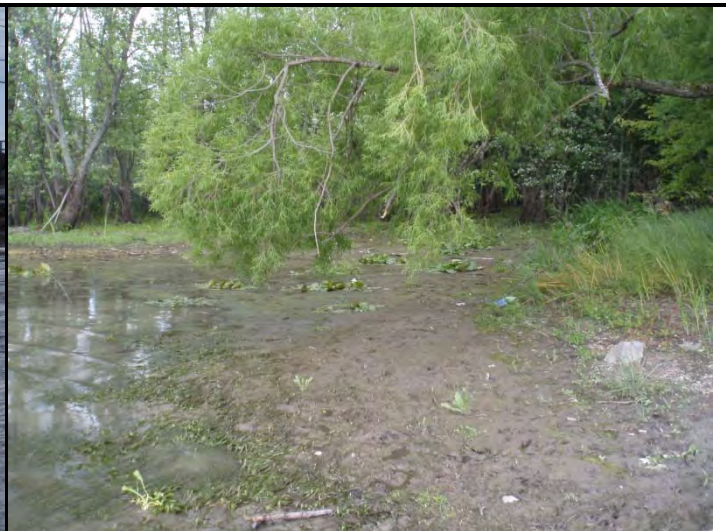
Photo 2. Evidence of flooding upstream of bridge
