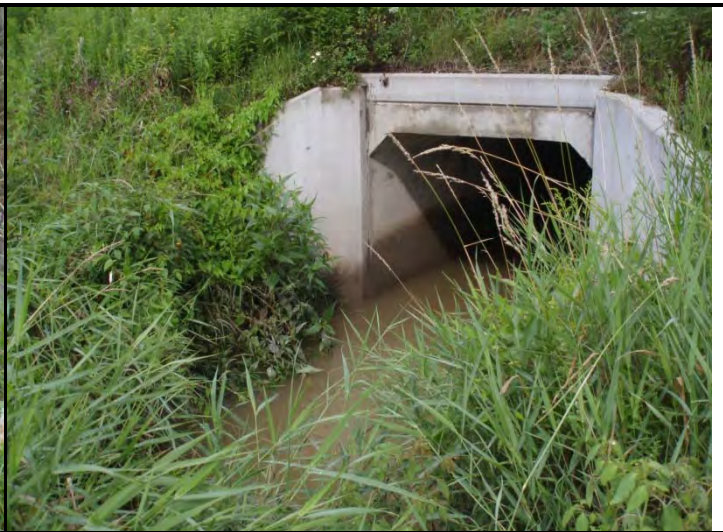
Photo 2. Upstream of bridge
