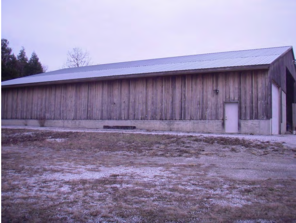
Figure 11. Town sand shed and adjacent gravel lot includes more than 0.5 acres of potentially treatable impervious surface.
