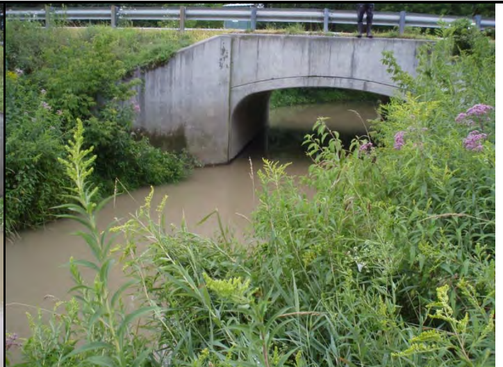
Photo 2. Upstream of bridge
