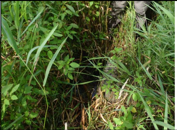
Photo 2. Downstream of culvert
