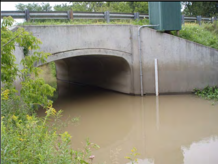
Photo 1. Downstream of bridge
