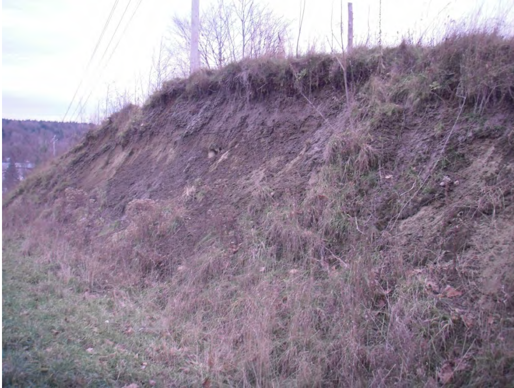
Figure 2. Oversteepened and eroding ditch backslope on west side of Durkee Rd. in Highgate Center.
