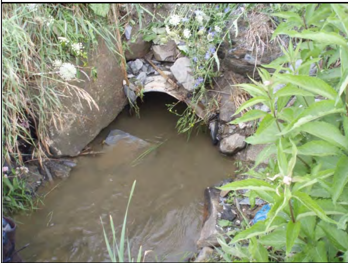
Photo 1. Upstream of culvert
