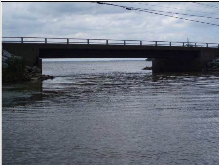
Photo 1. Route 7 bridge over the Rock River
