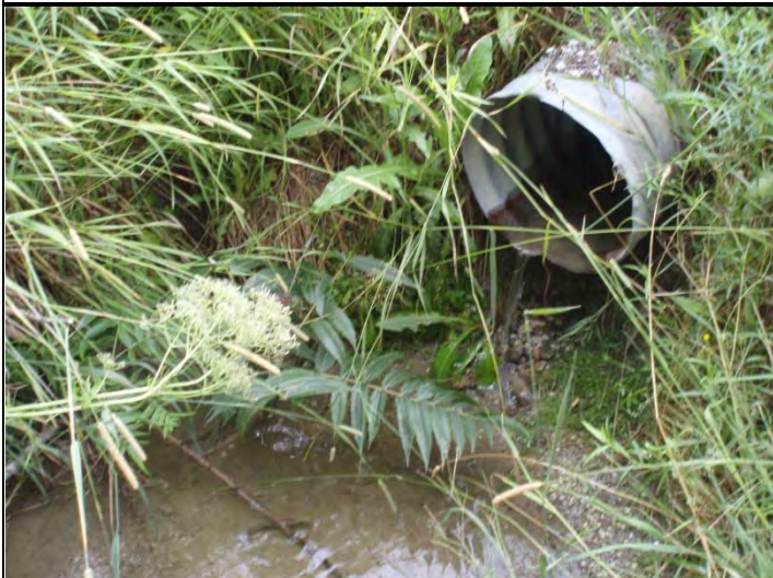
Photo 1. Downstream culvert
