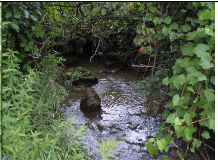
Photo 2. Downstream of culvert
