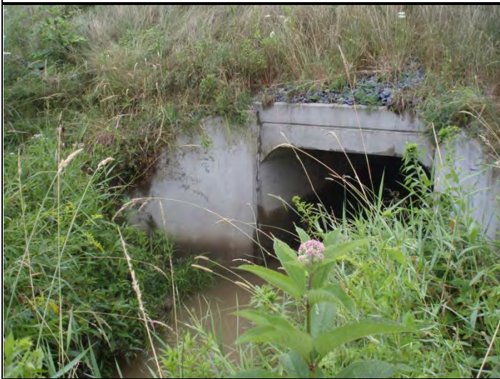
Photo 1. Downstream of bridge
