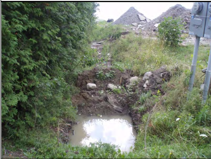
Photo 1. Potential culvert outfall area
