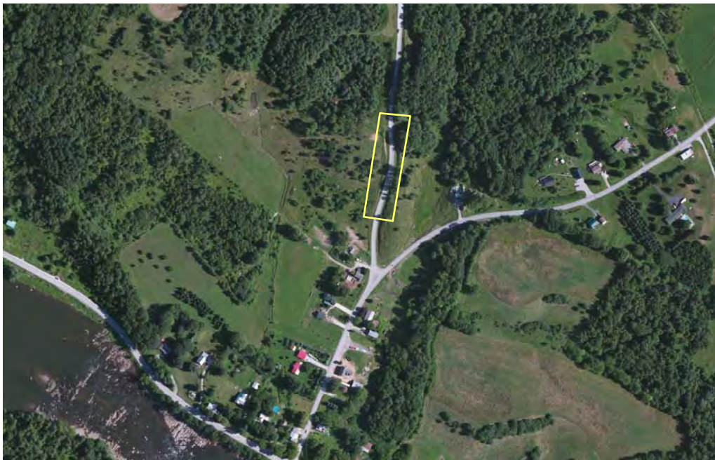
Figure 1. An area of eroding slopes along Durkee Road is highlighted in yellow.
