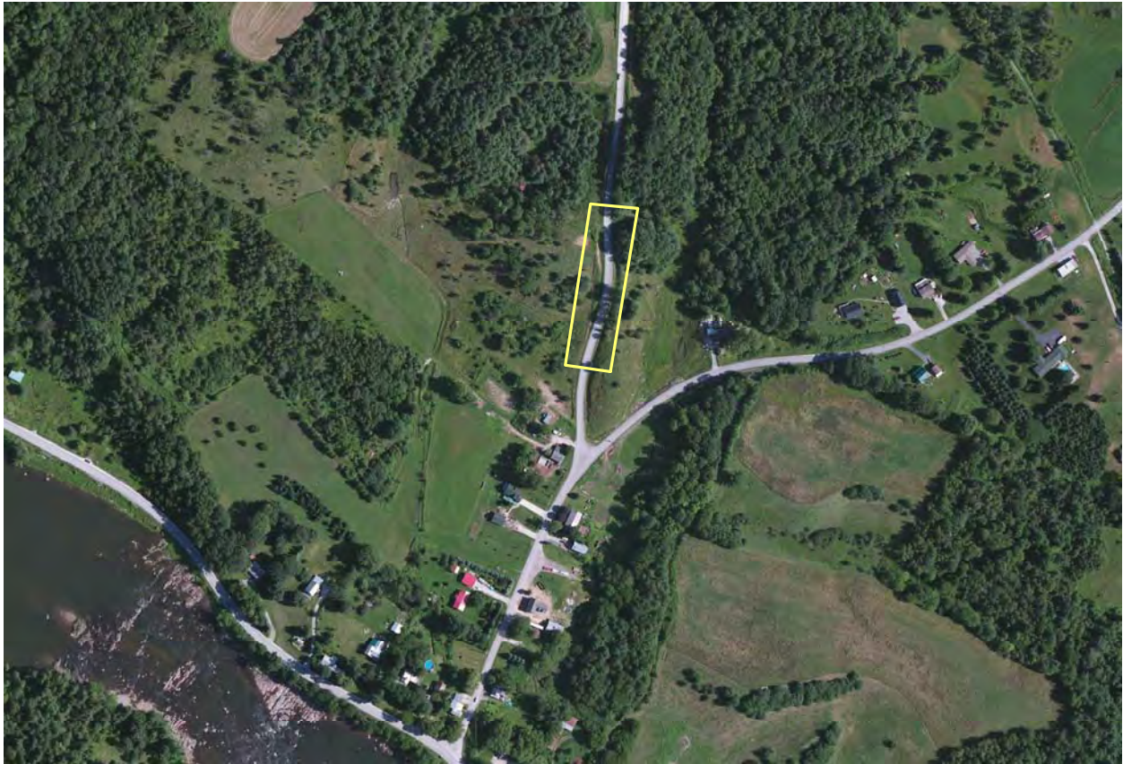
Figure 1. Area of eroding slopes highlighted in yellow.
