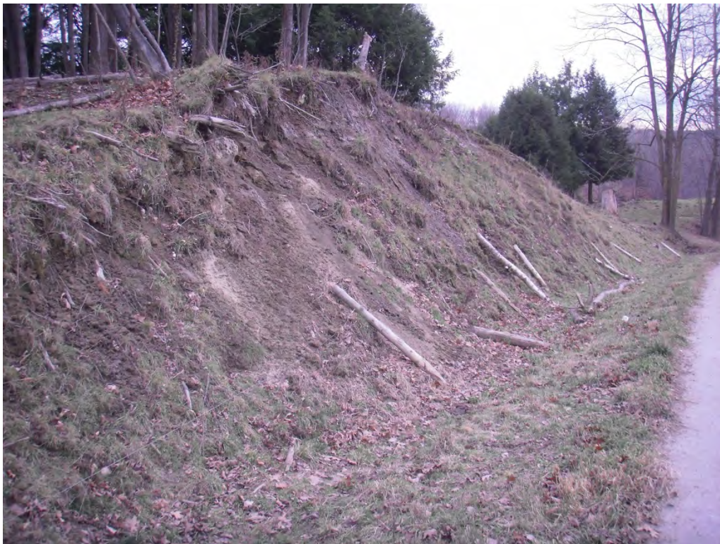
Figure 3. Eroding ditch backslope on the east side of Durkee Road in Highgate Center.
