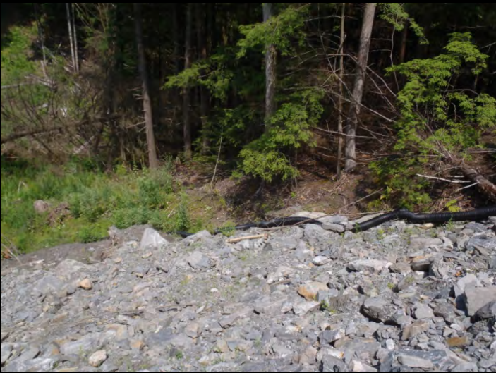
Photo 5. Pipe that now drains parking lot area
