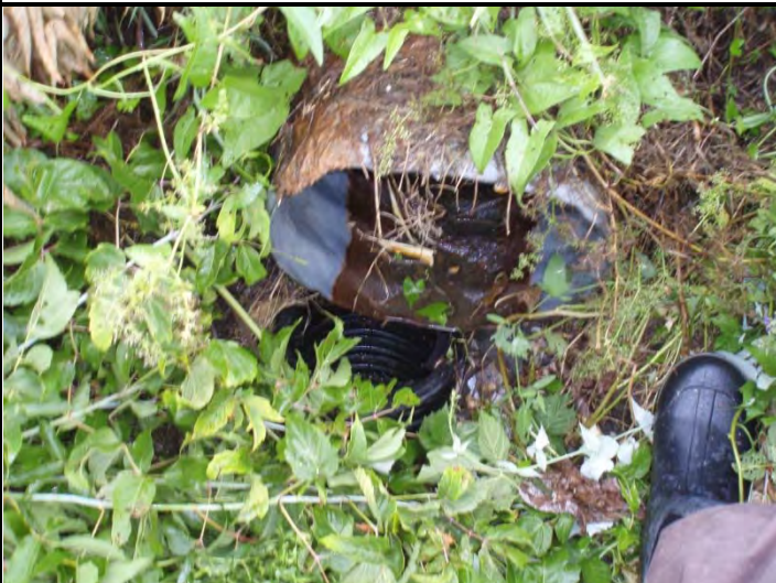
Photo 1. Downstream culvert drains to pipe
