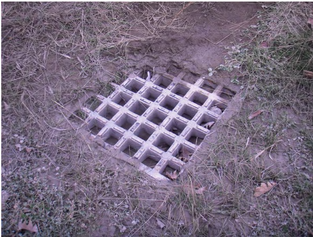
Figure 12. Sediment has completely filled catch basin at the Highgate town sand shed.
