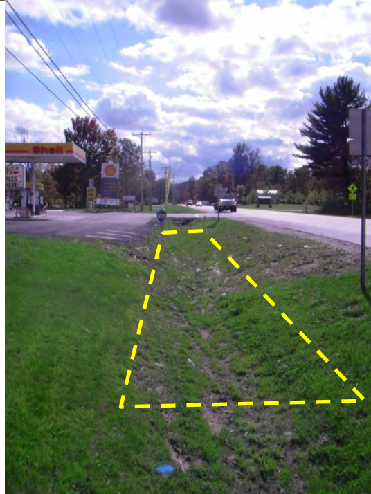
Figure 8. Looking south along the east side of Route 7 in front of the Georgia Market.
