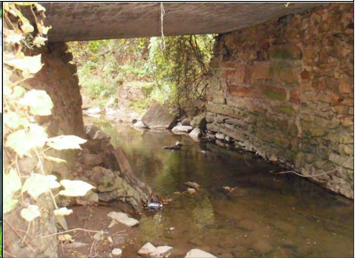
Photo 2. Falling rip-rap at outlet
