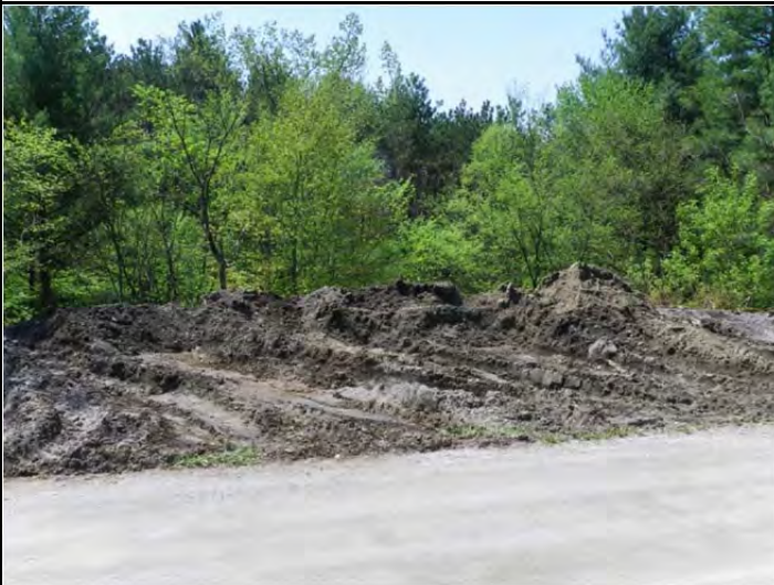
Photo 1. Fill on south-side of Decker Rd
