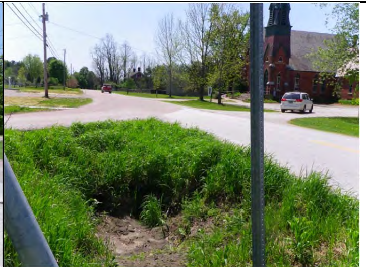
Photo 2. Sediment build up in the "Y" median
