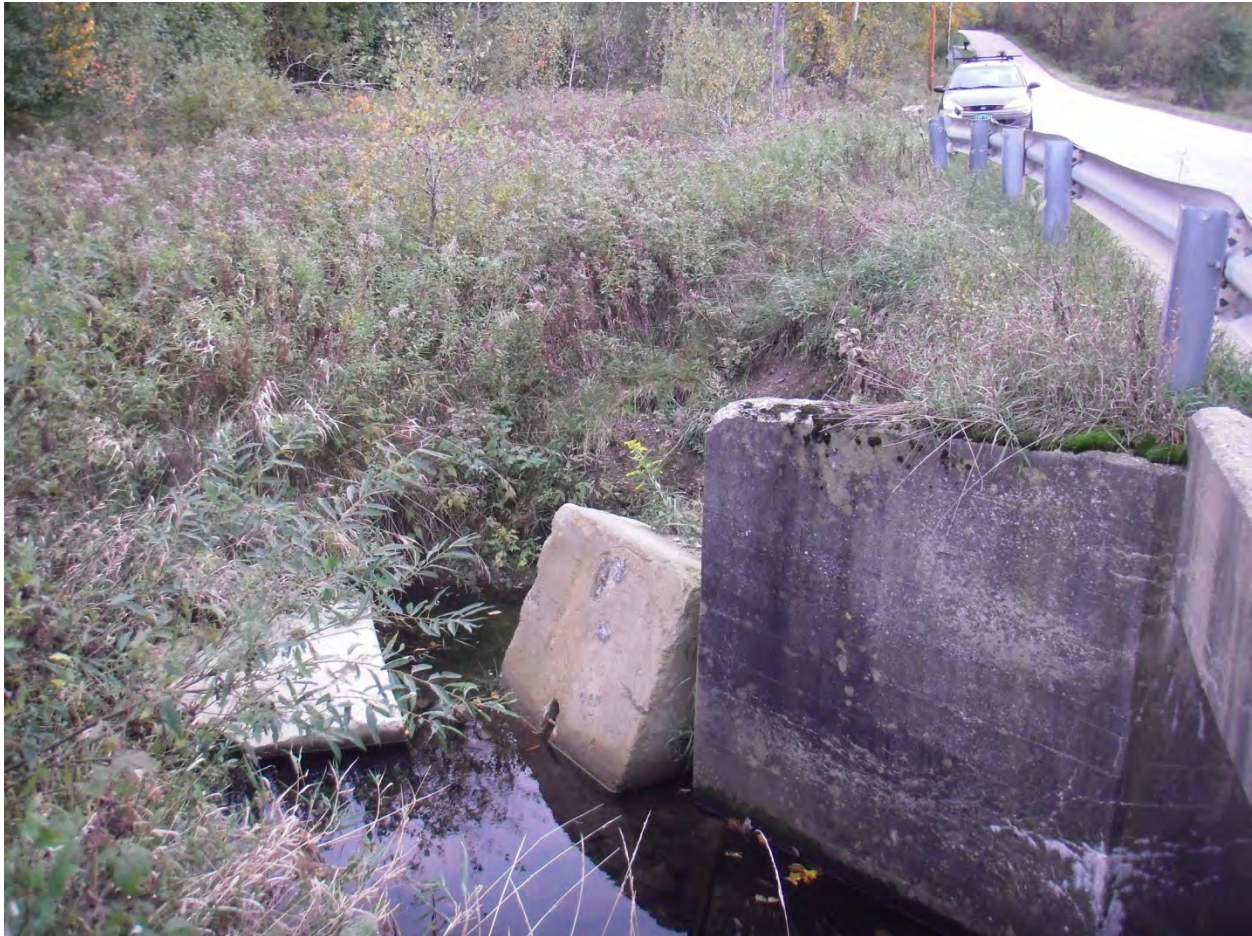
Figure 21. Failing slope near inlet to box culvert over Mill River on Oakland Station Rd.
