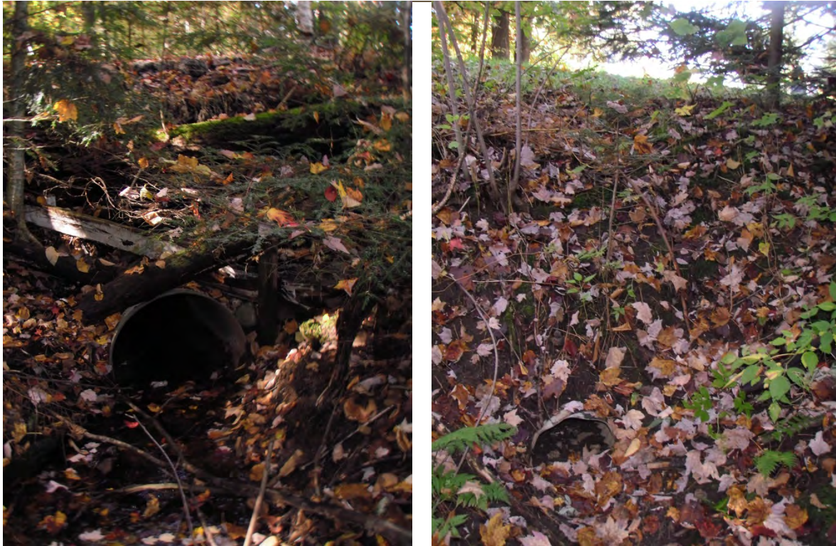
Figure 20. Partially clogged culverts with unstable cover slopes.
