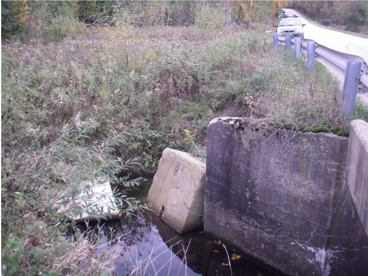
Figure 6. Failing slope near inlet to box culvert over Mill River on Oakland Station Rd.
