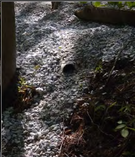
Photo 2. Recently repaired driveway
