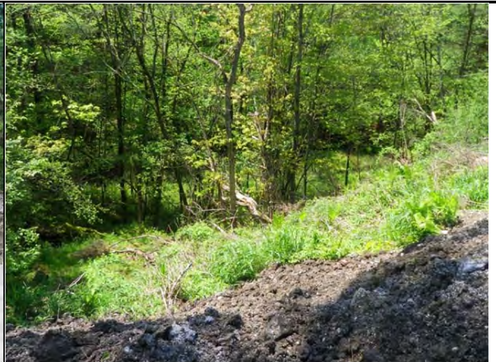
Photo 2. Natural area below placed fill
