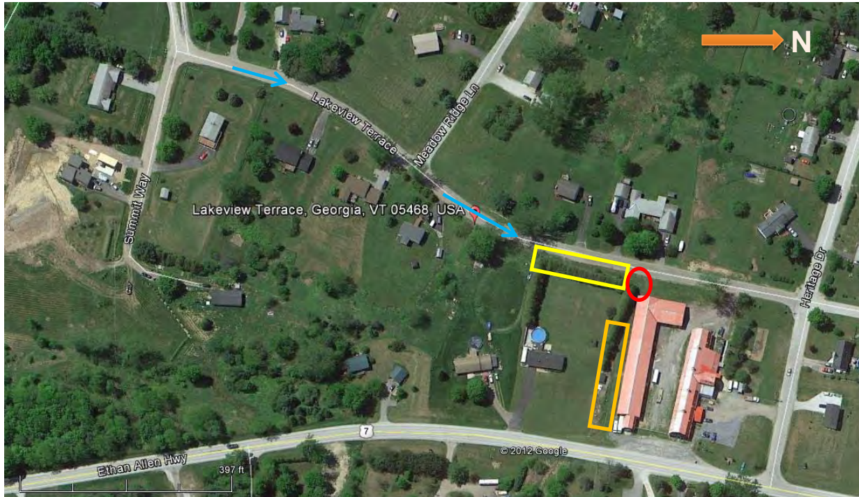
Figure 5. Red Barn property and surrounding neighborhood. Location of existing scour hole shown in red. Potential STP locations shown in yellow and orange.
