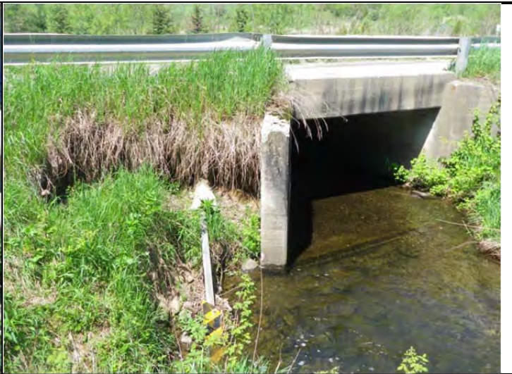
Photo 2. Looking downstream at bank erosion
