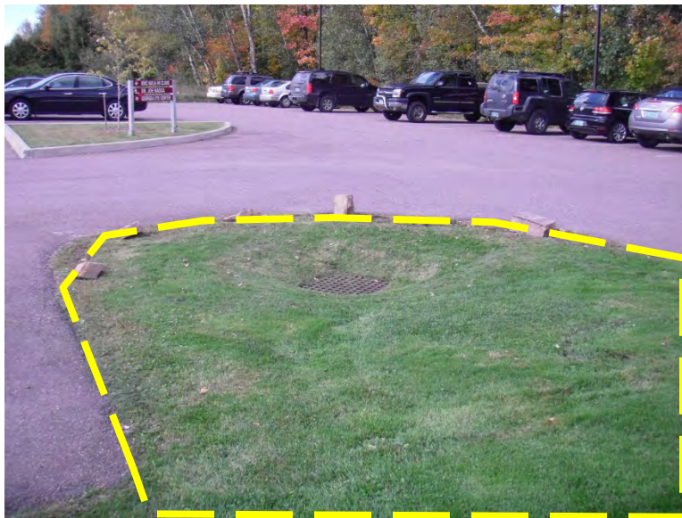
Figure 4. Existing catch basin that could be retrofitted and integrated into a stormwater treatment practice.
