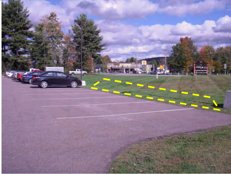
Figure 3. Catch basin is located beneath red pickup truck in the photo. Stormwater from half of parking lot could be routed to lawn area shown right half of photo.
