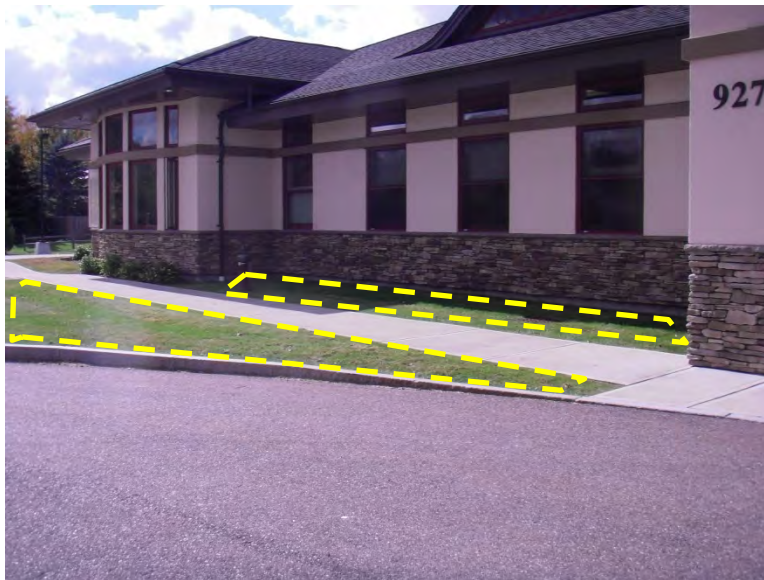
Figure 2. Example of area where roof runoff could be routed to a rain garden.
