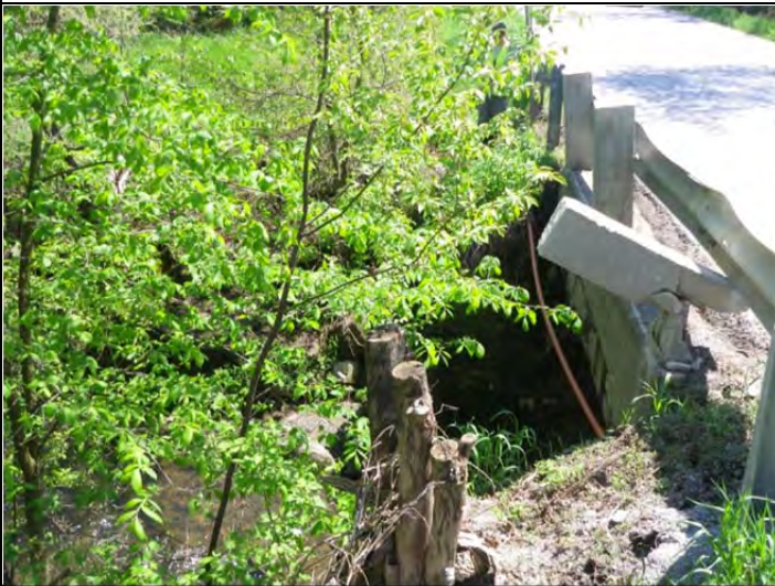
Photo 1. Erosion caused by road runoff
