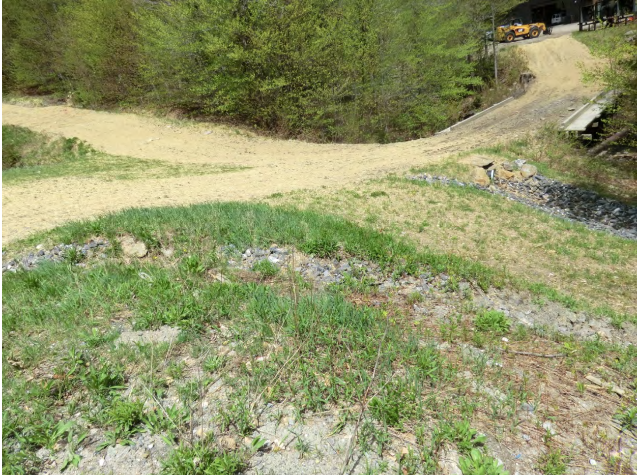
Figure 21. Erosion control and stormwater management improvements in vicinity of Snowplant Work road, photo taken May 13, 2013 by Mary Nealon of BCE.
