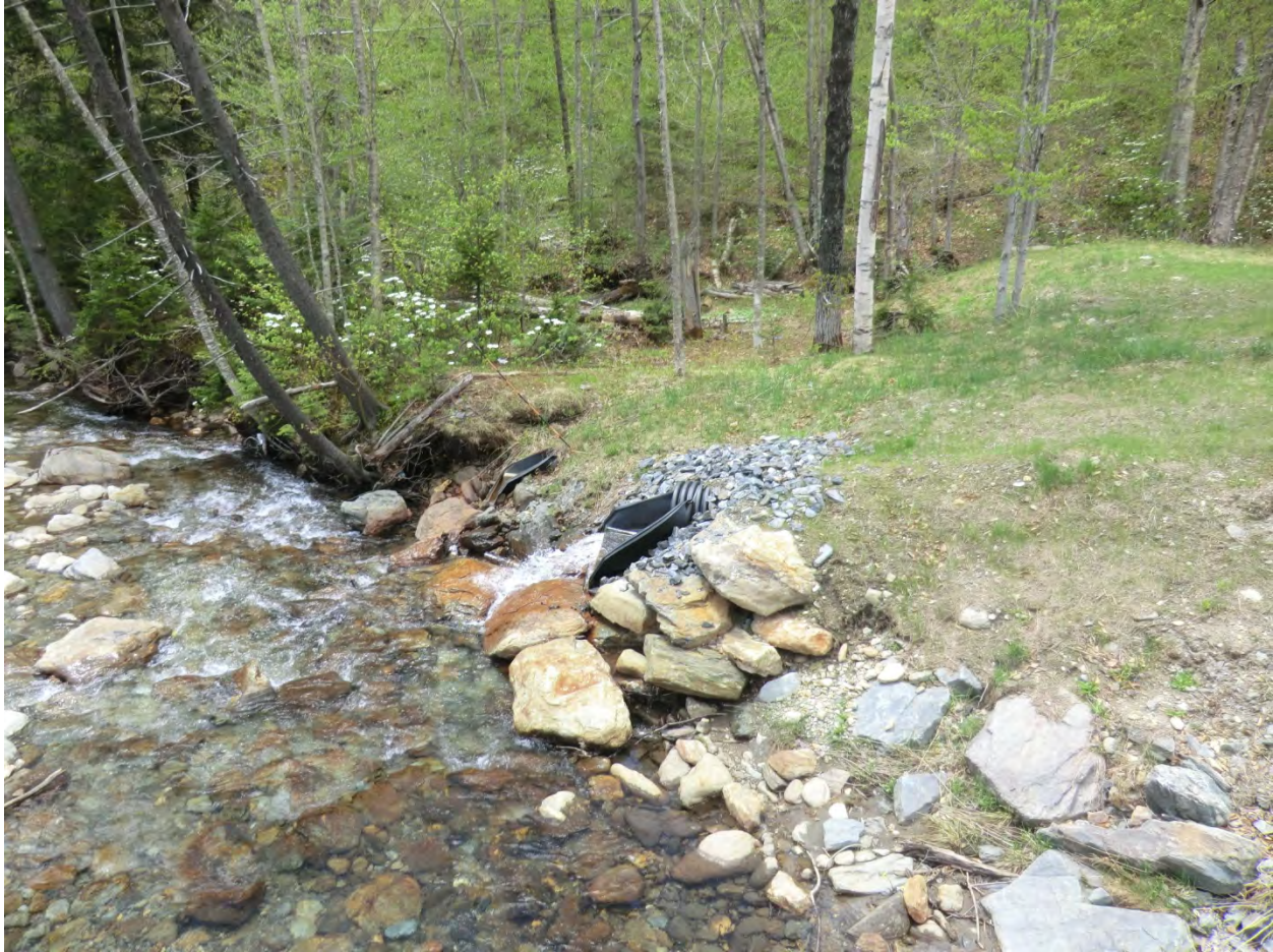
Figure 22. Separation of on mountain stream run-off and stormwater at Mansfield Exit; photo taken on May 13, 2013, by Mary Nealon of BCE.
