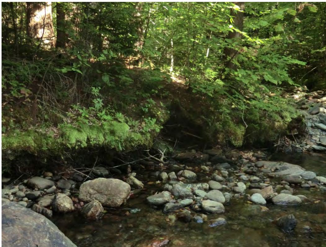
Figure 30. West Branch RM 6.5. had bank erosion at the downstream end (9/16/12)
