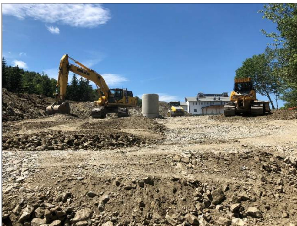
Photograph #7. Backfilling and compaction of processed blast rock from Long John Ski Trail at Lot E in the vicinity of DMH-120 and DMH-121, 07/02/2019.
