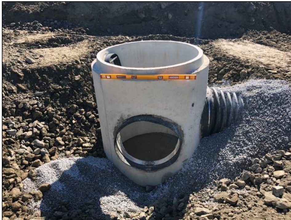
Photograph #6. Backfilling of crushed limestone at Lot E in the vicinity of DMH-121 for new 30-inch HDPE culvert installation, 06/27/2019.
