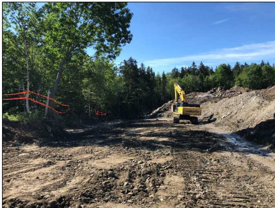
Photograph #5. Excavated soils being removed from Lot E for on-mountain soil disposal areas, 07/02/2019.
