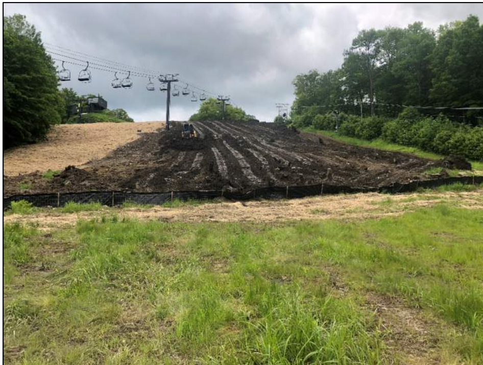
Photograph #4. Soil Disposal Area #8 receiving excavated soils removed from Lot E for use in regrading Sundance Ski Trail; completed portions stabilized with seed and hay mulch, 06/19/2019.
