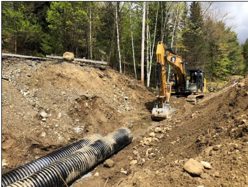
Photograph #2. New 24-inch HDPE culvert installation at south entrance to Somerset Road; swale to be lined with low permeability liner, 05/24/2019.
