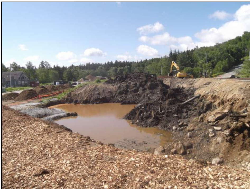
Photograph #1. Initial excavation for Carinthia Base Lodge, showing previously buried organic materials and iron-rich water, 06/28/2019
