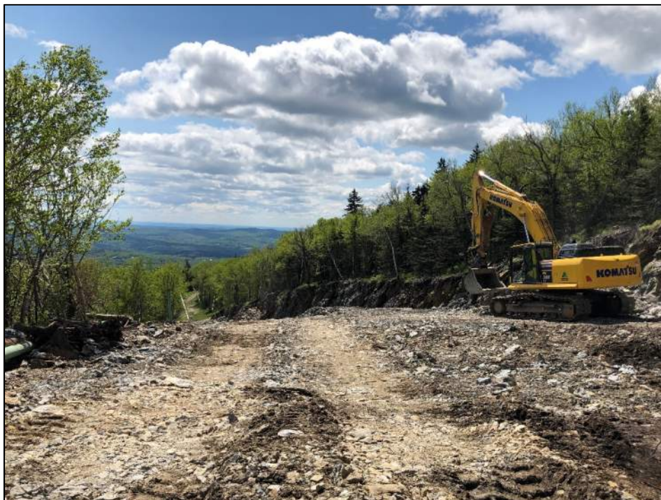
Photograph #3. Blast rock being removed from Long John Ski Trail for use as backfill during Lot E construction, 06/04/2019.
