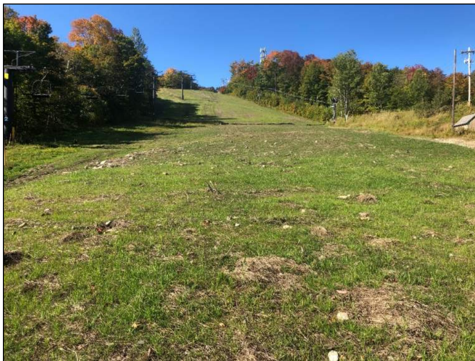
Photograph #9. Soil Disposal Area # 8 on regraded Sundance Ski Trail, nearing permanent stabilization, 09/27/2019.
