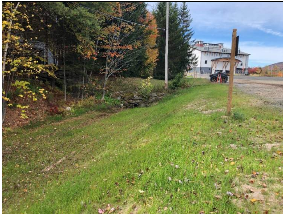
Photograph #10. Reshaped swale with low permeability liner completed along west side of Lot E, 10/08/2019.
