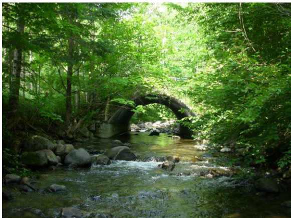
Figure 64. Turkey Hill Rd. stream crossing in reach T1.07 is undersized but is an excellent design for fish and other aquatic organism passage.
