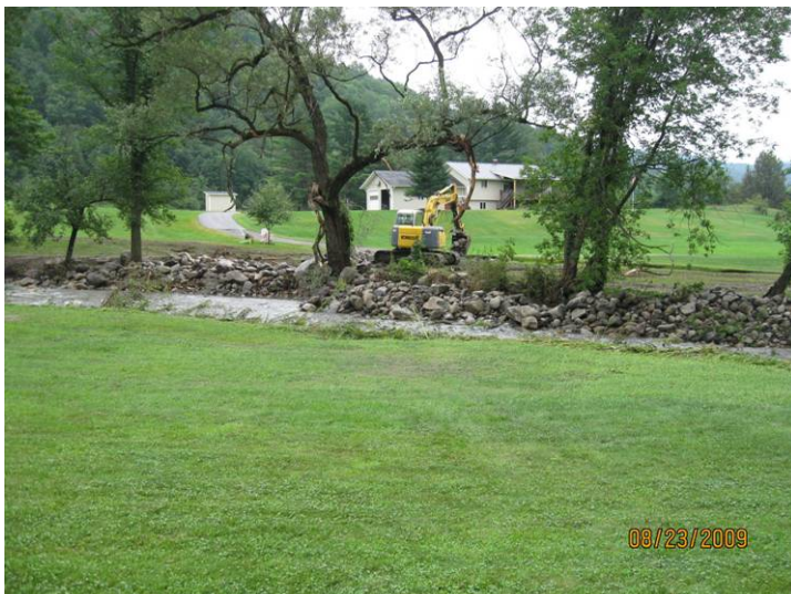
Figure 17. Windrowing of sediments following flash flooding, particularly upstream of undersized bridges and culverts and similar constrictions, is not uncommon and is frequently undocumented. This can complicate understanding channel evolution and the movement of sediment in a stream system.
