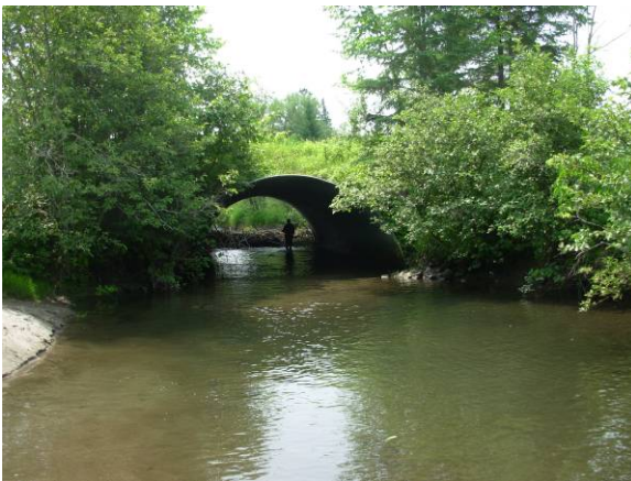
Figure 66. Arch culvert at Dearborn Hill Rd. in segment T1.09A is partially obstructed by a beaver dam just upstream of the inlet
