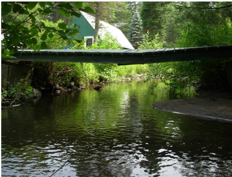
Figure 69. Development encroachment in segment T1.09C; bank toe stabilization placed on both banks; bridge is a channel constriction with some deposition noted upstream
