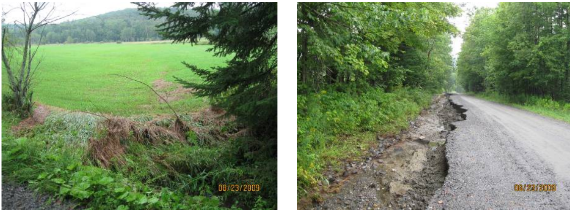
Figure 15. The field swale at left contributed sufficient water in a heavy downpour to initiate gullying along the road (right), eventually combining with a tributary downhill to wash out a 6 ft. culvert and a section of the road.
