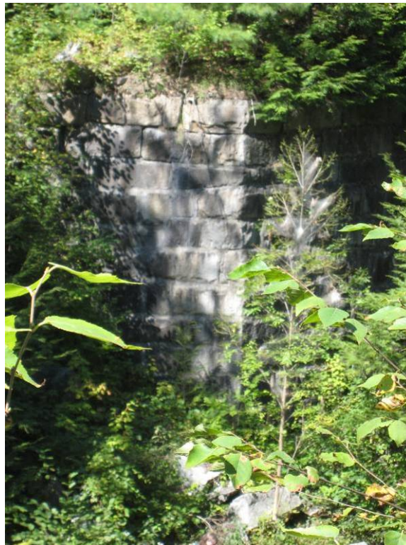
Figure 28: Wells River mainstem, Reach M04, old railroad bridge abutment.
