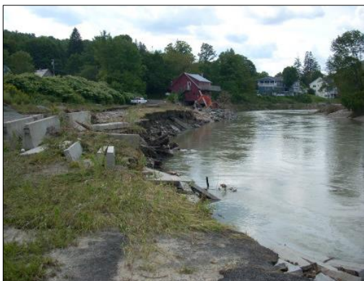
BEFORE – Eroding and degraded floodplain, Ottauquechee River. Photo credit: M. Caduto, VTDEC
