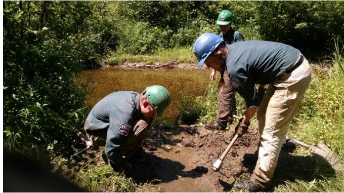
VYCC crews dig drainage ditches to allow standing water to drain from the roadway.
