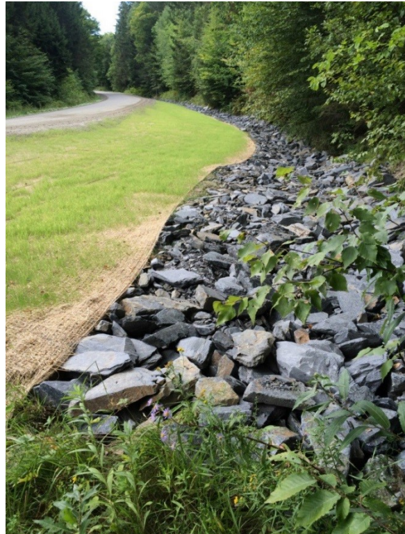
AFTER – Ditch was properly sloped and rock-lined to slow water velocity and five feet of the road shoulder was vegetated, leaving trees undisturbed.
