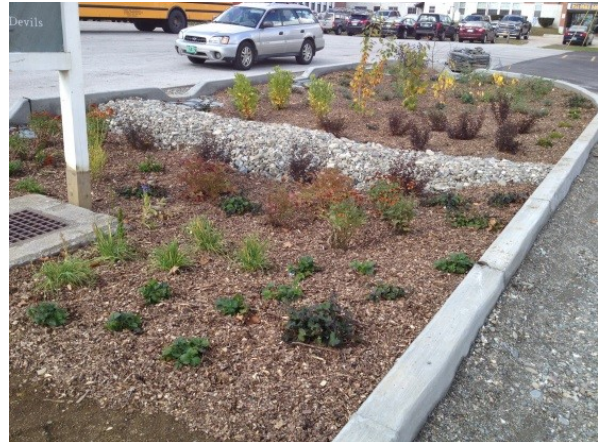
AFTER – Three bioretention/rain garden areas installed to treat stormwater runoff (above and below).
