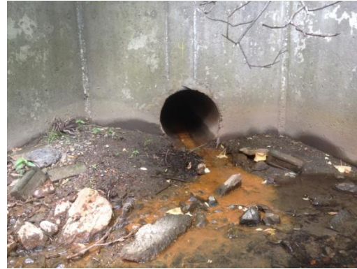
Figure 5: Outfall 24 on June 5th, 2012.
