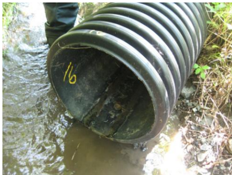
Figure 27: Outfall T16 on June 7 th , 2012.
