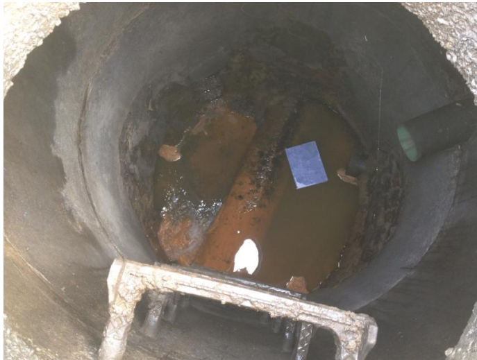
Figure 35: TL-3 Storm Manhole on October 25th, 2012.
