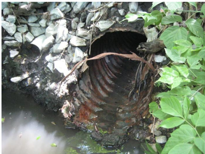
Figure 31: Outfall T123 on June 7th, 2012.
