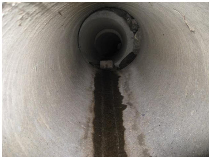
Figure 23: View Looking up Outfall 15 on August 27 th , 2012 (Disconnection in pipe visible 10 ft up pipe from outfall)
