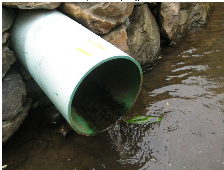
Figure 25: Outfall 11 on June 4th, 2012
