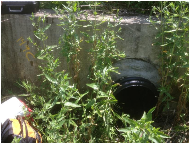
Figure 33: Outfall T149C; Slight trickle observed on June 20 th , 2012.
