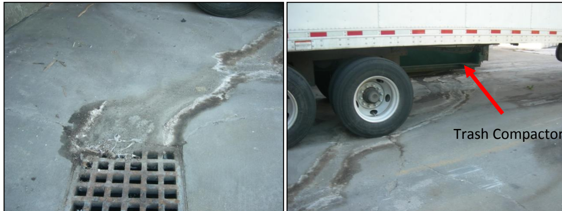
Figure 29: T16.CBA, located in Hannaford Loading Dock. Seepage from trash compactor evident on June 21 st , 2012.
