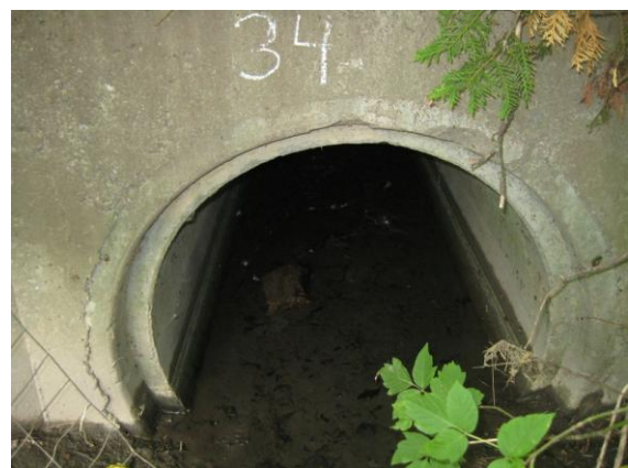
Figure 13: Outfall 34 on June 6th, 2012
