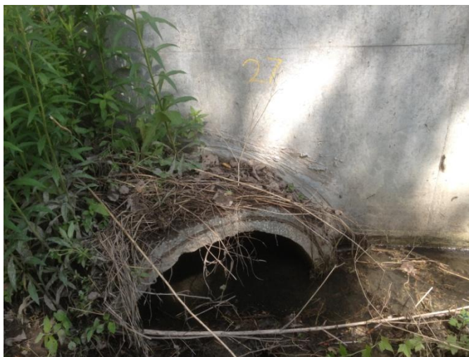
Figure 11: Outfall 27 on June 6th, 2012.
