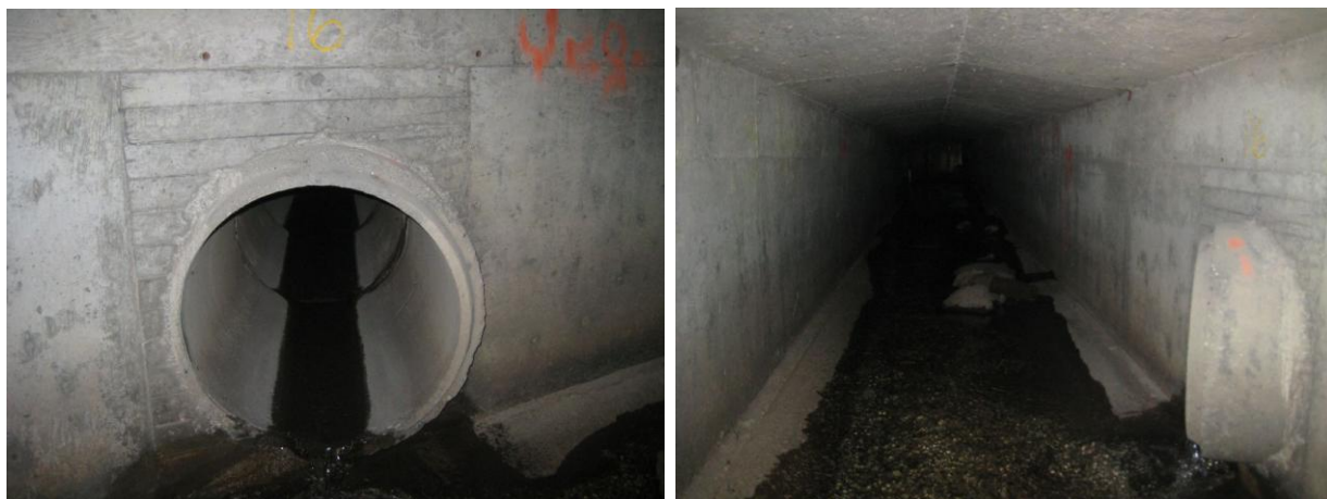
Figure 20: Left - Outfall 16 on June 5th, 2012, Right- Side View of Outfall 16 Looking Through Culvert Under Upper Welden St./Main St.
