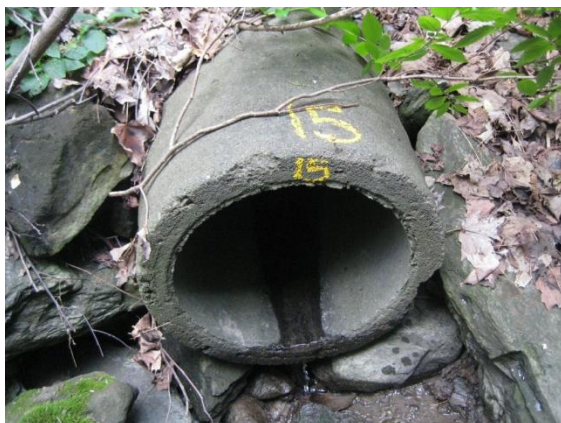
Figure 22: Outfall 15 on June 5th, 2012.
