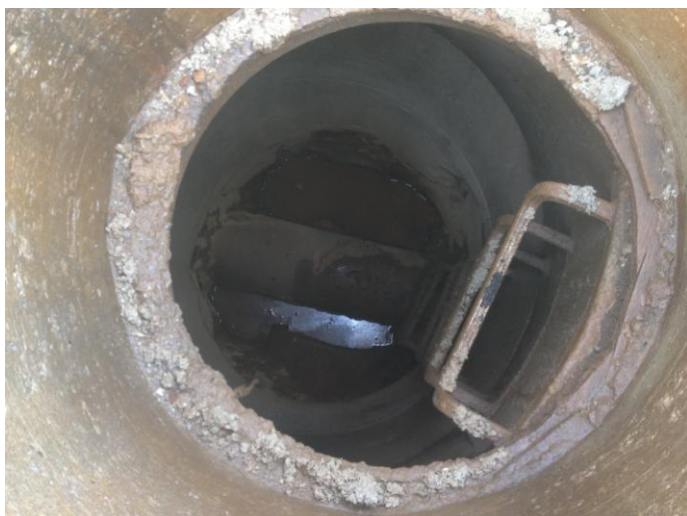
Figure 36: Structure TL-5 on October 25th, 2012.
