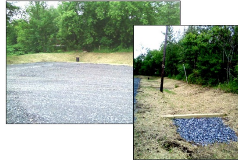
Figure 1: Infiltration Gallery
