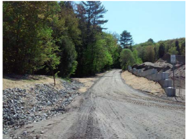
Road within town garage sand pit area upgraded to include stabilized ditches, roadside turnouts with settling pools, road crown and waterbars
