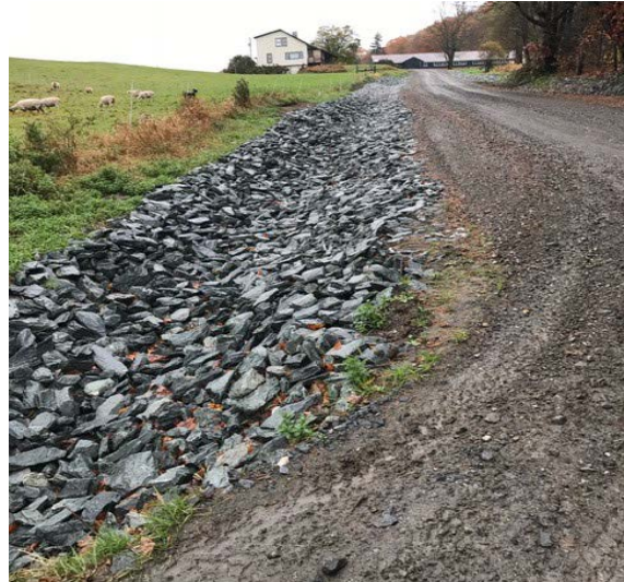
The same road in Corinth, VT after rock lining ditches, crowning the road and applying other BMPs to meet standards.
