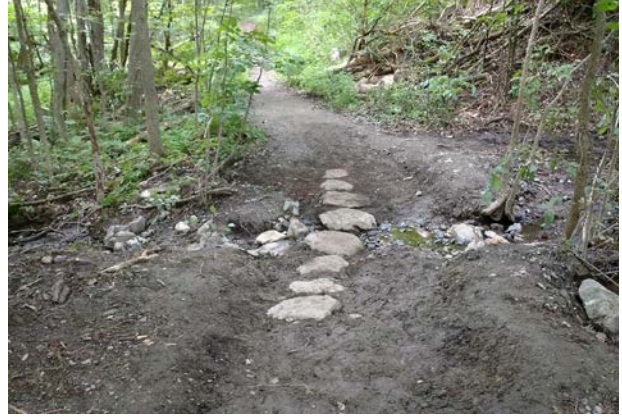
After regrading, several rock weirs were placed downstream to slow water velocity and steppingstones added where the old culvert had been
