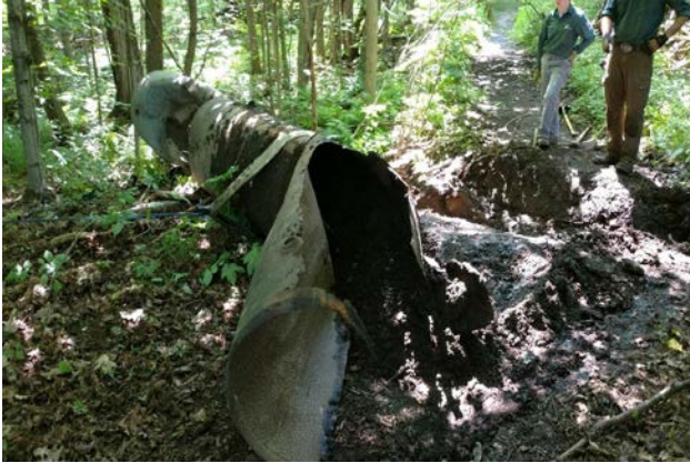
Decades old culvert that was preventing natural flow of the river was removed
