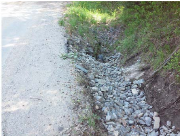
Stone lined ditches at the town garage site with check dams to slow velocity
