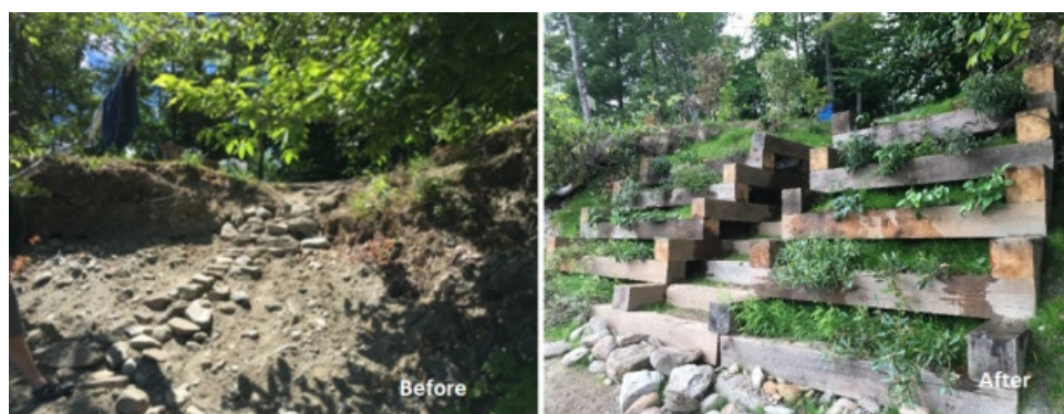
Figure 5. Live Crib Wall project, before and after, built to stabilize this eroding shore along Waterbury Reservoir State Park. Live Crib Walls are built from natural materials, like these untreated hemlock timbers and native plants.
