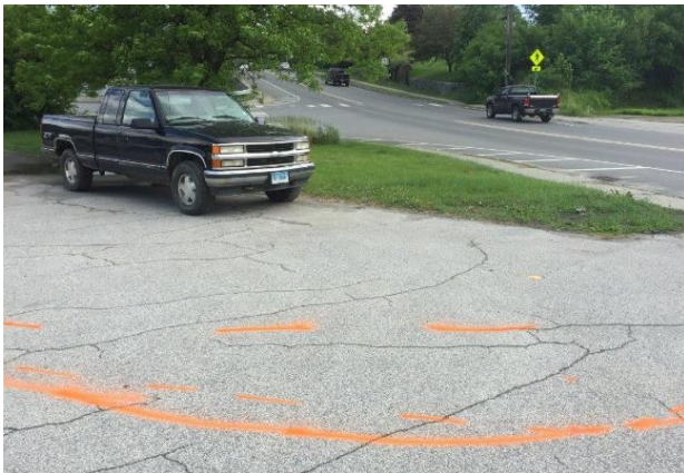
Figure 26. Before (top) and after (bottom) installation of bioretention system on Center Street in Northfield, completed by Central Vermont Regional Planning Commission
