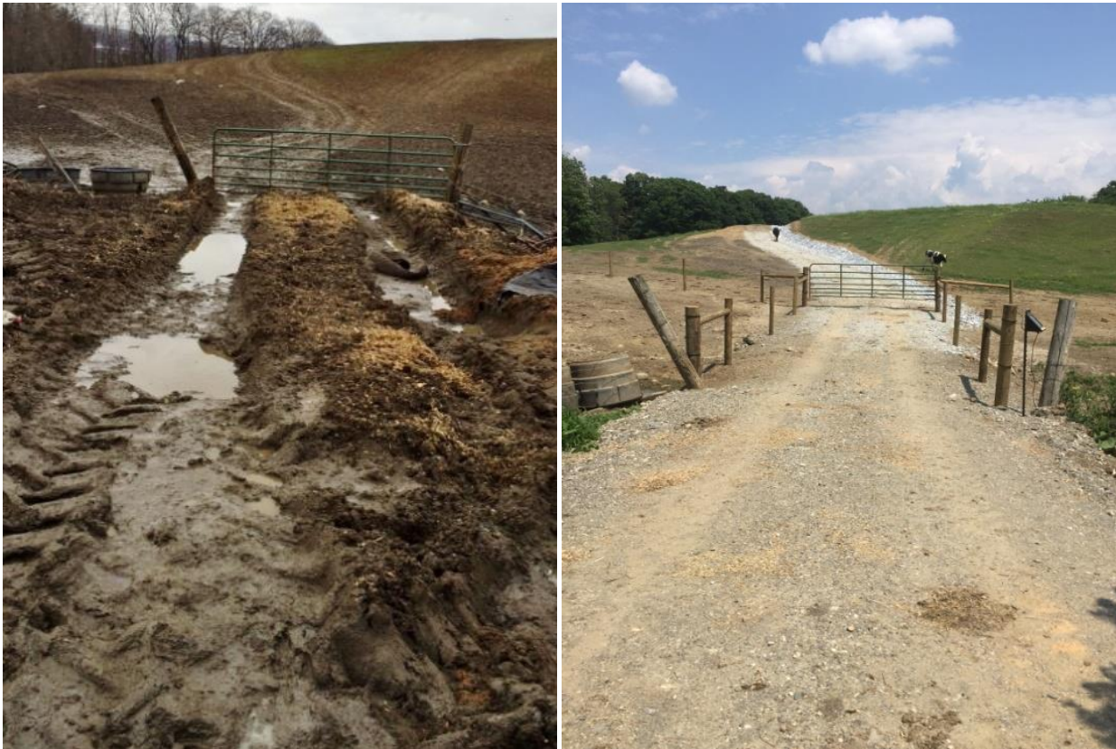
Figure 21. Before (left) and after (right) installation of livestock exclusion fencing and improved laneway and water crossing, completed by Poultney Mettowee Conservation District with ANR funding
