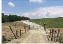
Livestock exclusion fence and improved laneway completed by Poultney Mettowee Conservation District (see Figure 21)
