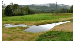
Bioretention system on Morey Road, Hyde Park completed by Lamoille County Conservation District (see Figure 27)
