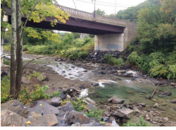
Randolph Dam removal completed by the White River Partnership (see Figure 25)
