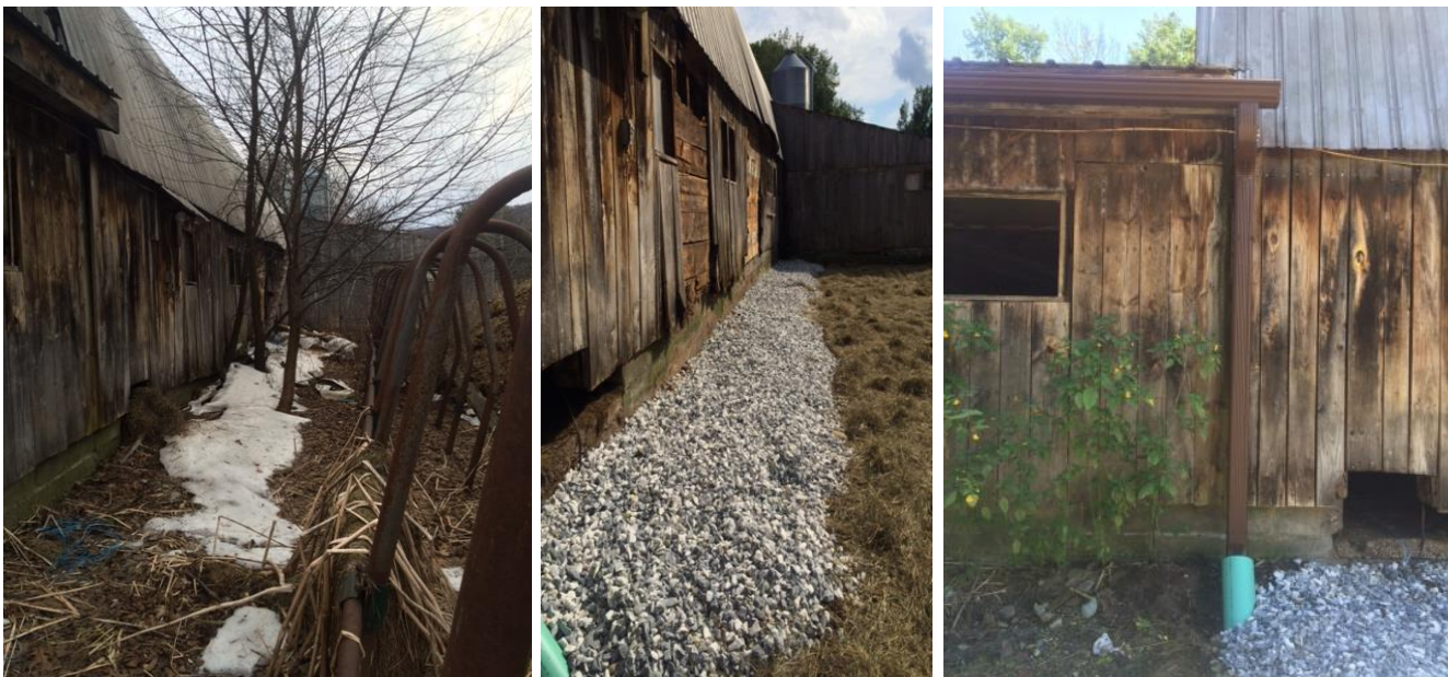
Figure 22. Before (left) and after (middle and right) installation of barnyard roof runoff diversion practices, completed by Poultney Mettowee Conservation District with ANR funding
