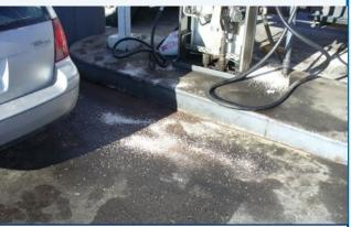
Even though absorbent material was placed on the spilled diesel fuel, the fuel flowed off the concrete pad because the employee did not surround the spill with absorbent material. Remember: first surround the spill with absorbent material, then cover it!
