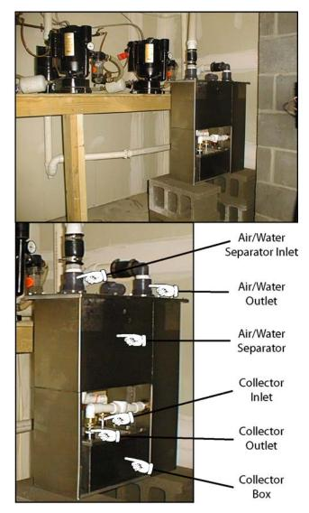
Pilot Installations: Two RME2000 amalgam separators were installed and observed in the pilot.
