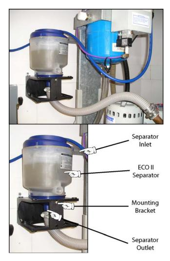
both the separator and collection tank, the entire unit is removed and replaced when full. Removal is simple: disconnect the upper hose and pour the provided disinfectant into the inlet. Seal the inlet with the provided plug. Disconnect the lower hose and seal with the provided plug. Remove the entire unit from its mounting bracket and ship to the mercury recycler using the shipping materials provided in the recycling kit.
