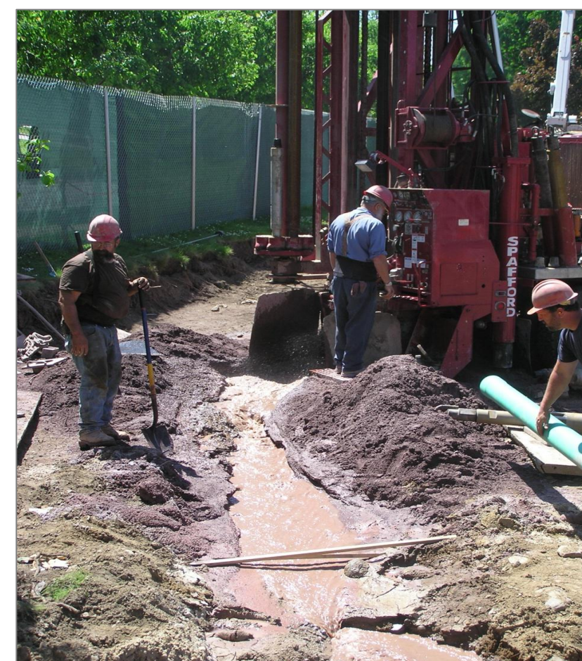
Figure 14. Drilling in the Monkton Fm at Champlain College for a standing column (shallow) geothermal system.
