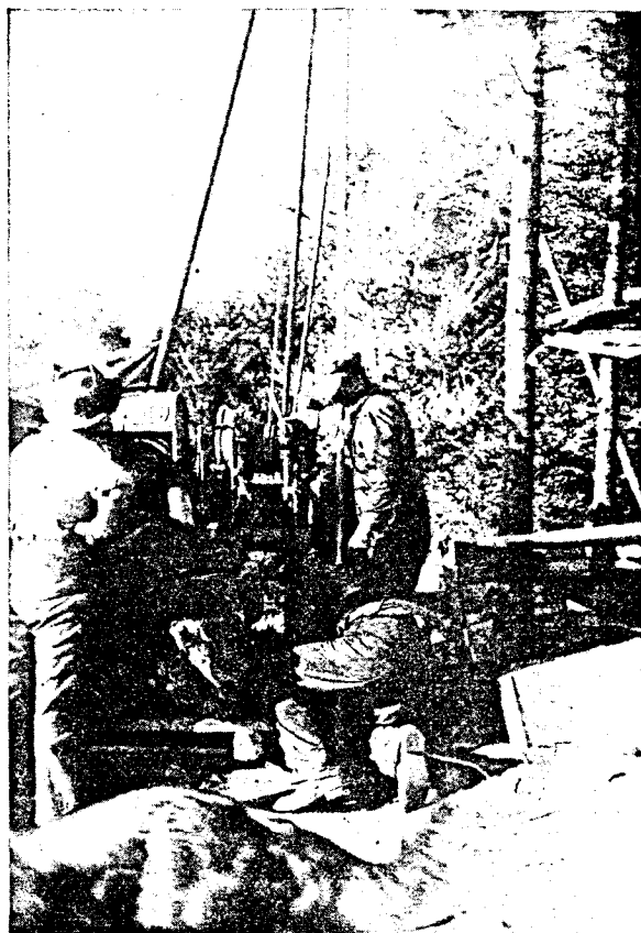
Drilling at Cuttingsville
