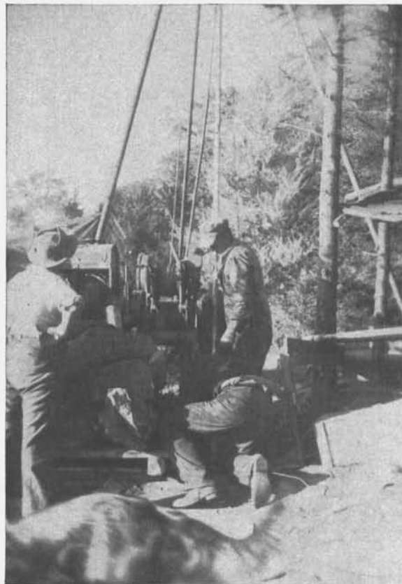
Drilling at Cuttingsville
