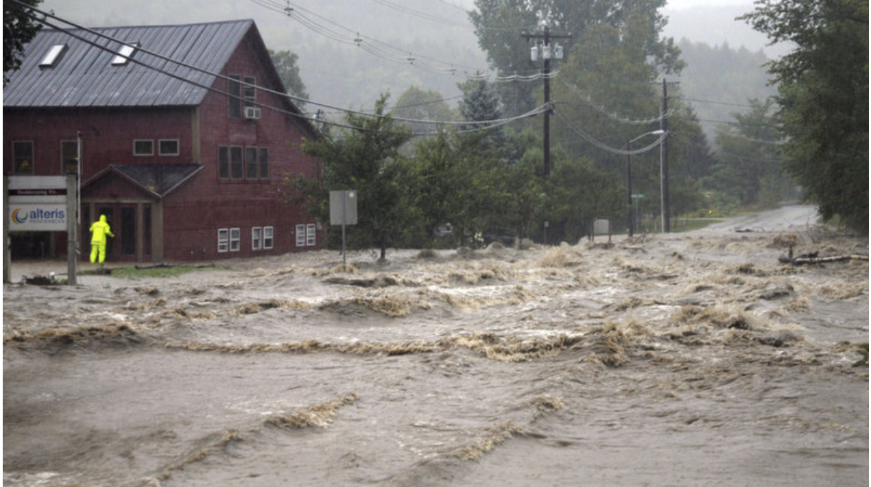
A Washed Out Road in Waitsfield, VT after Tropical Storm Irene in 2011 (Sandy Macys, AP Photo)
