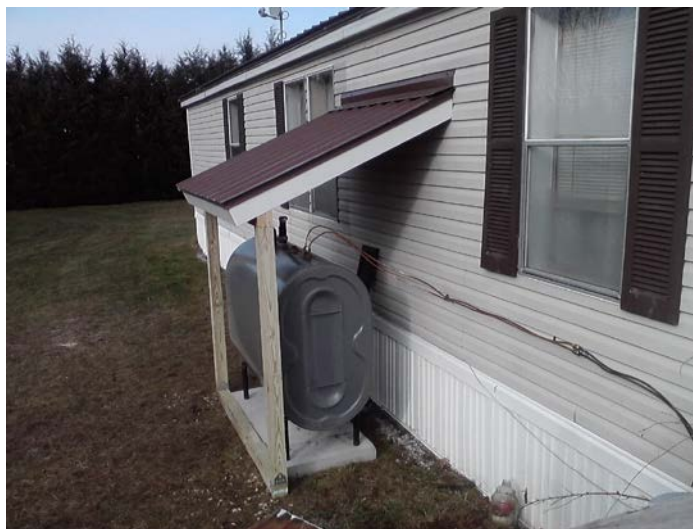
2012 AST installation showing concrete pad and roof
