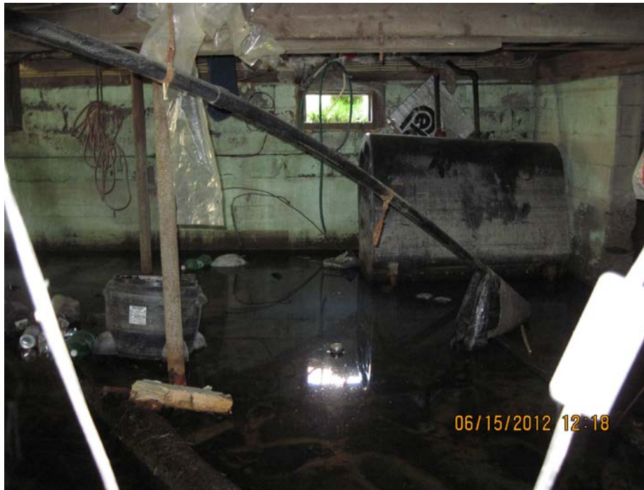
AST release caused by Tropical Storm Irene, Roxbury, VT
