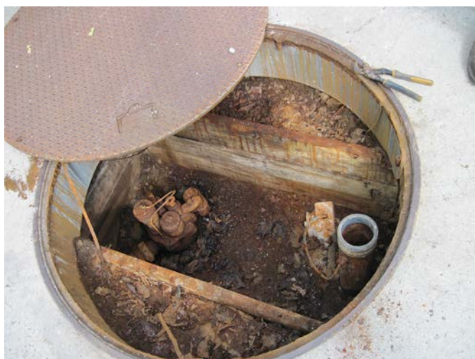
Single-walled UST system without secondary containment and the number of these tanks in VT
